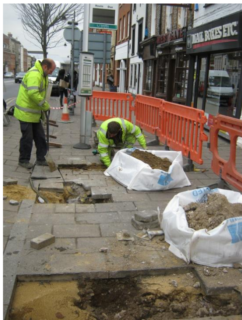
Plate 1: general view of work in progress
