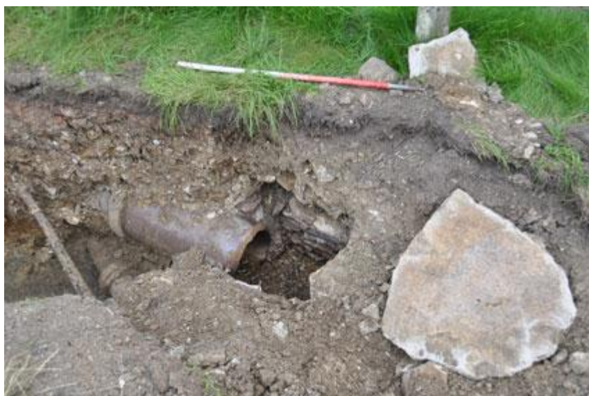
Plate 8: Modern alterations to the 18 th century stream culvert 5/9.
