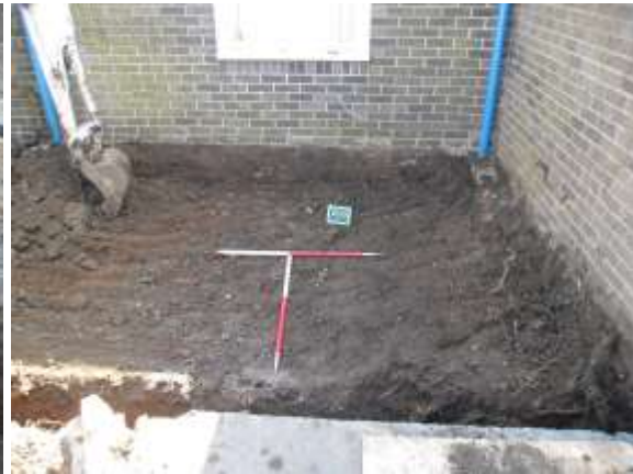
Plate 2. Reduction of platform inside foundation trenches
