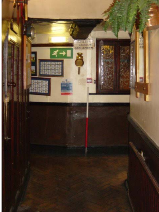
Plate 6: The Office wall showing remnant of spine beam and later angled alteration to create access to kitchens
