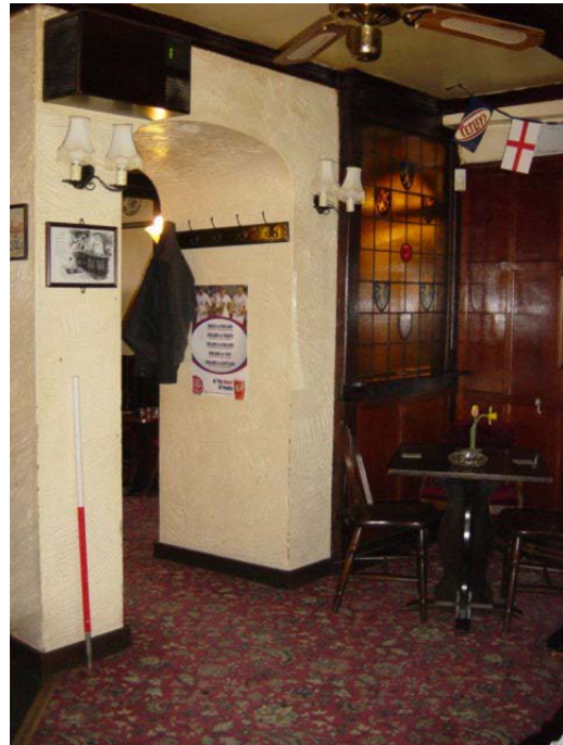
Plate 1: The arch created when fireplaces were removed and adjacent 20th century inserted glass panel
