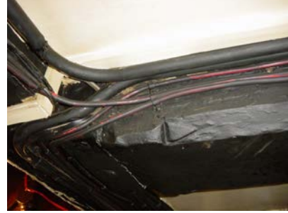
Plate 7: Detail of the chamfer-stop at the end of the spine-beam, this would have marked the original end of the room now shortened by the insertion of the late partition wall
