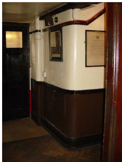
Plate 2: Rear of partition shown abutting earlier wall remnant and drainpipe.
