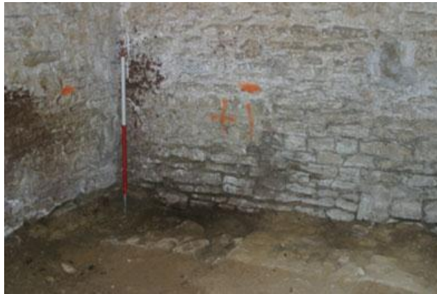
Figure 11. Wall 402, with mortar lintel (403) and stone blocking (404)
