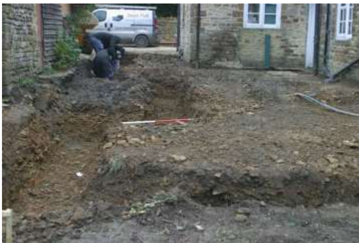
Plate 3: Eastern view of site
