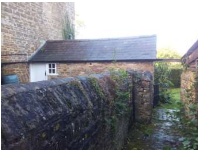
Plate 1: Western view of outbuilding
