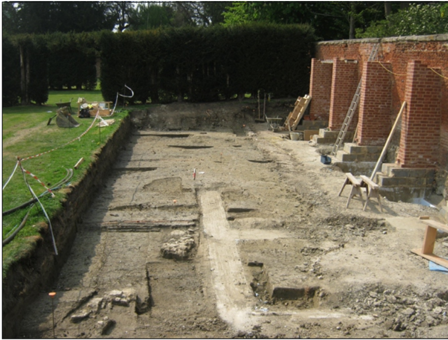
Figure 4. Site photograph; looking west.
