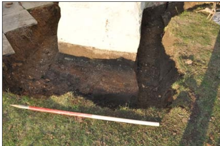
Plate 2. South west buttress on tower
