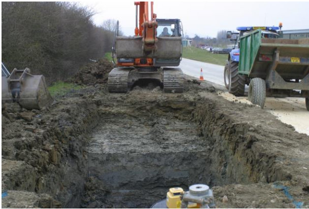
Plate 1: Sceptic tank trench
