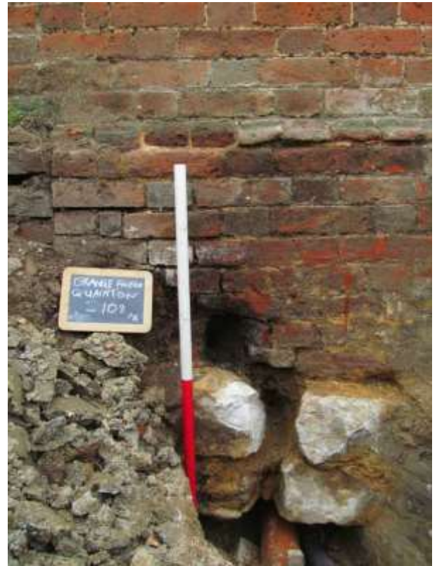
Plate 5. Section S.108, Building B4 foundations.
