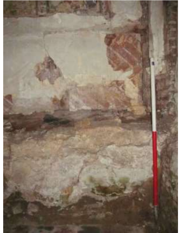
Plate 7. Wall between Building B2b & B2d
