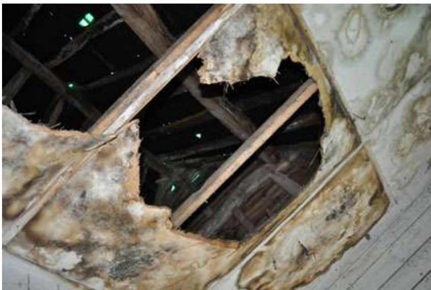
Plate 2 Unit S1 view of the end gable roof truss
