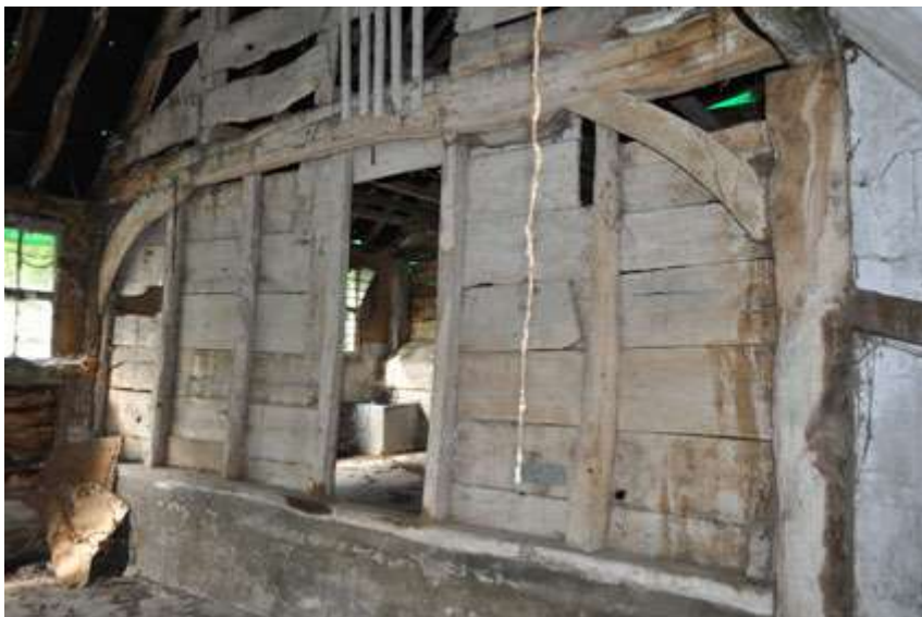
Plate 6 Timber frame between units S4 and S6
