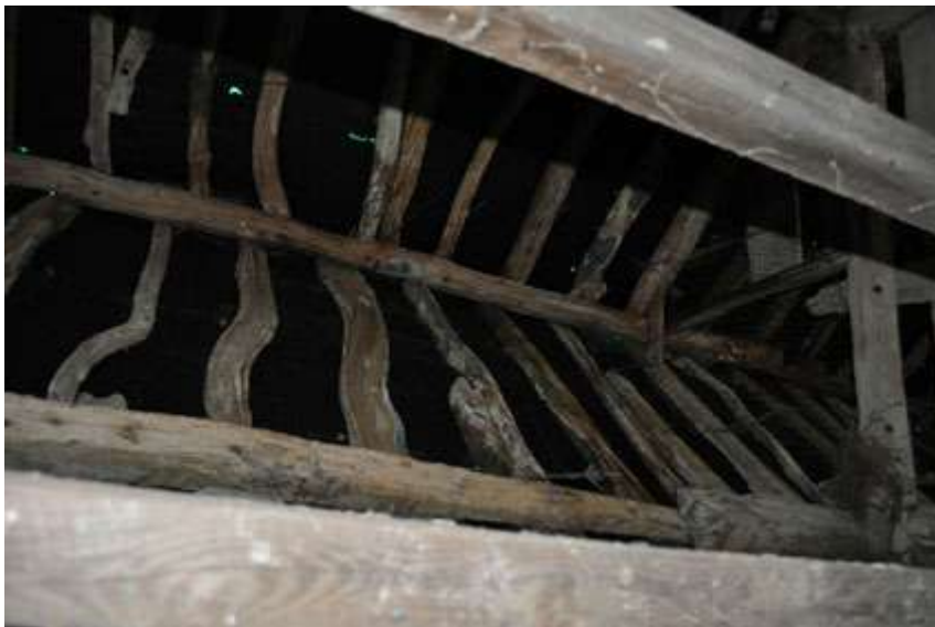
Plate 8 Common rafters and ridge beam
