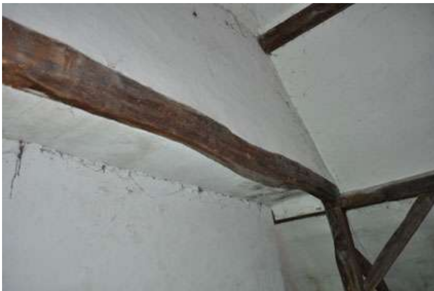
Plate 4 Unit S3 part of the timber structure
