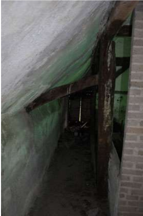
Plate 9 Braces in north aisle
