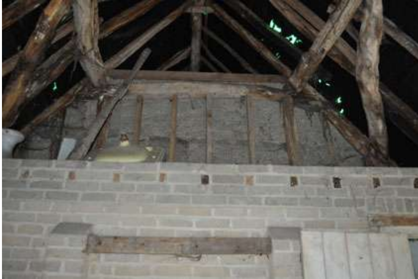
Plate 5 Truss between units S3 and S4
