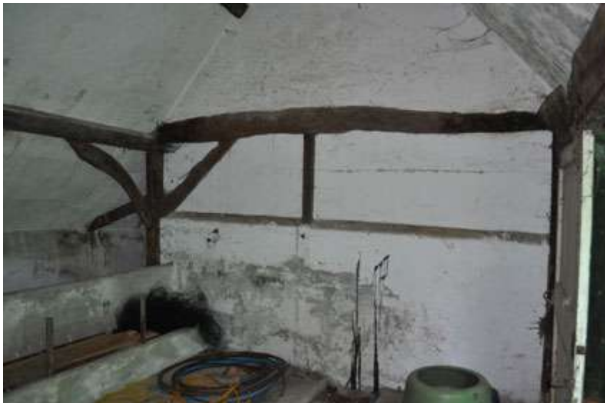
Plate 3 Unit S3 part of the timber structure
