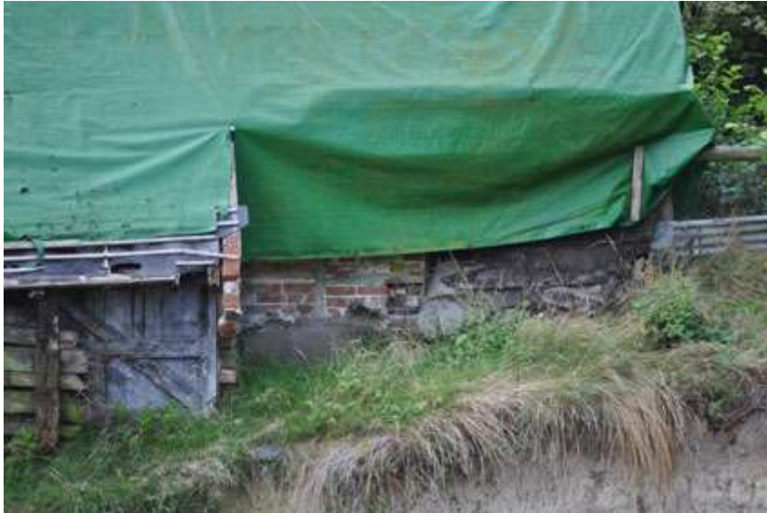
Plate 1 Timber framing and brick infill wall in north wall
