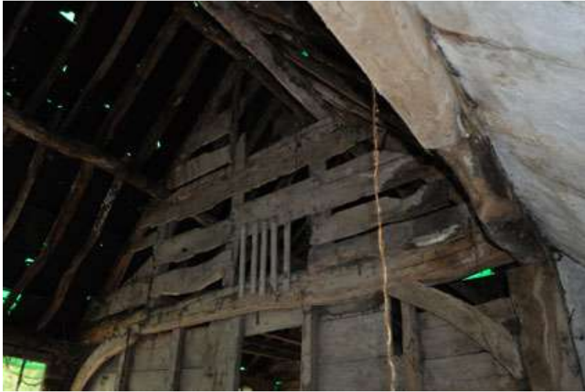
Plate 7 Timber Truss between units S4 and S6
