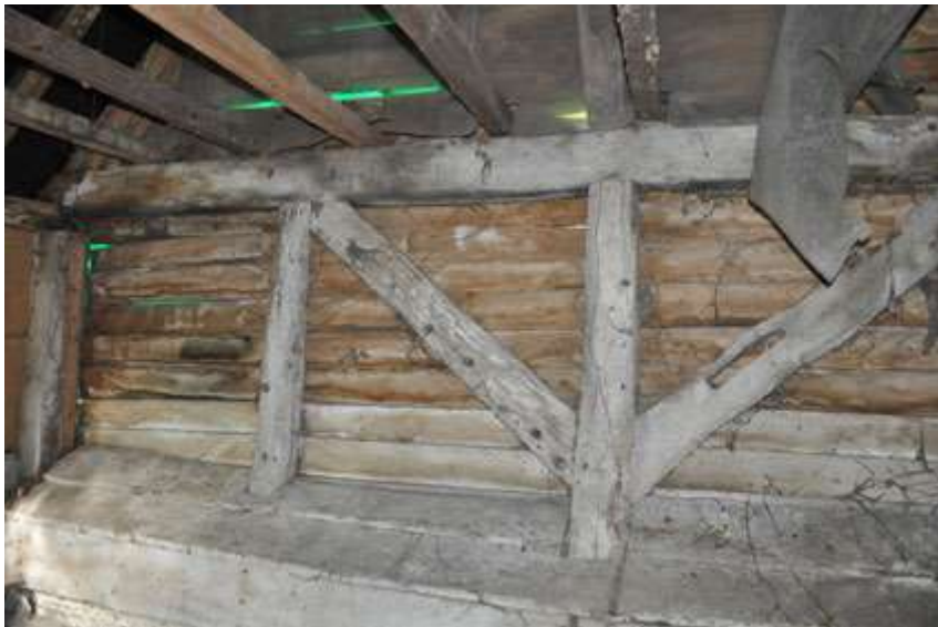
Plate 10 Timber frame in west wall
