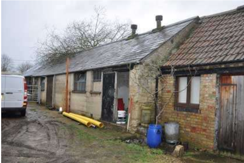
Plate 1 Northern range central block, a reworked cow-shed
