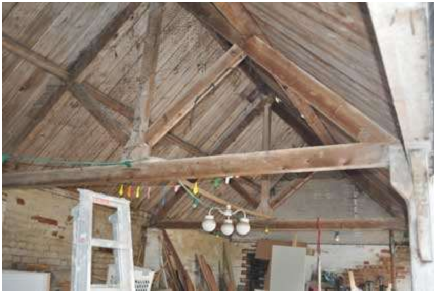
Plate 4 Trusses in eastern part of North range
