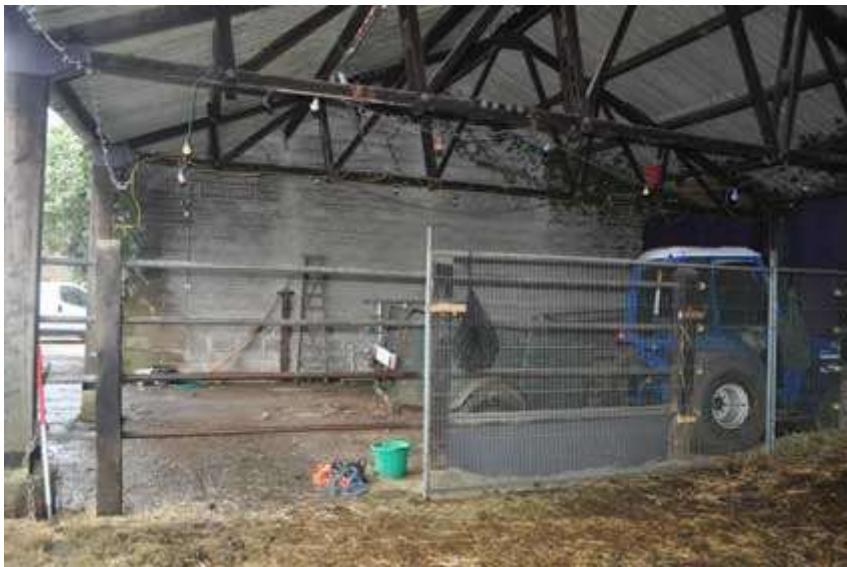
Plate 10 Interior of south building
