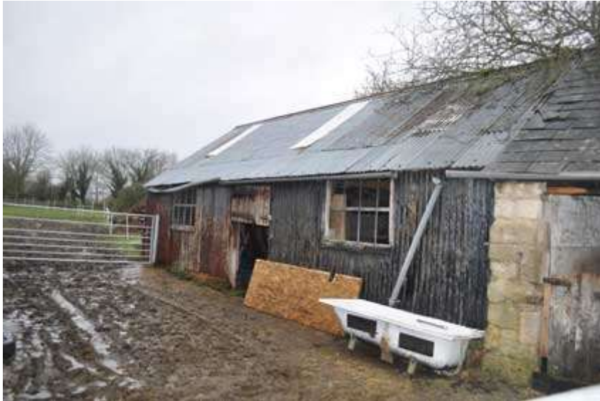
Plate 5 North range, west end of south façade
