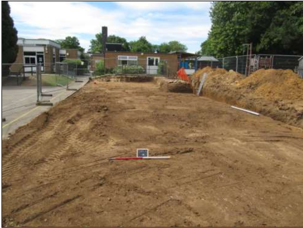
Plate 2: Site after ground reduction and excavation of footings trench 1, looking west.
