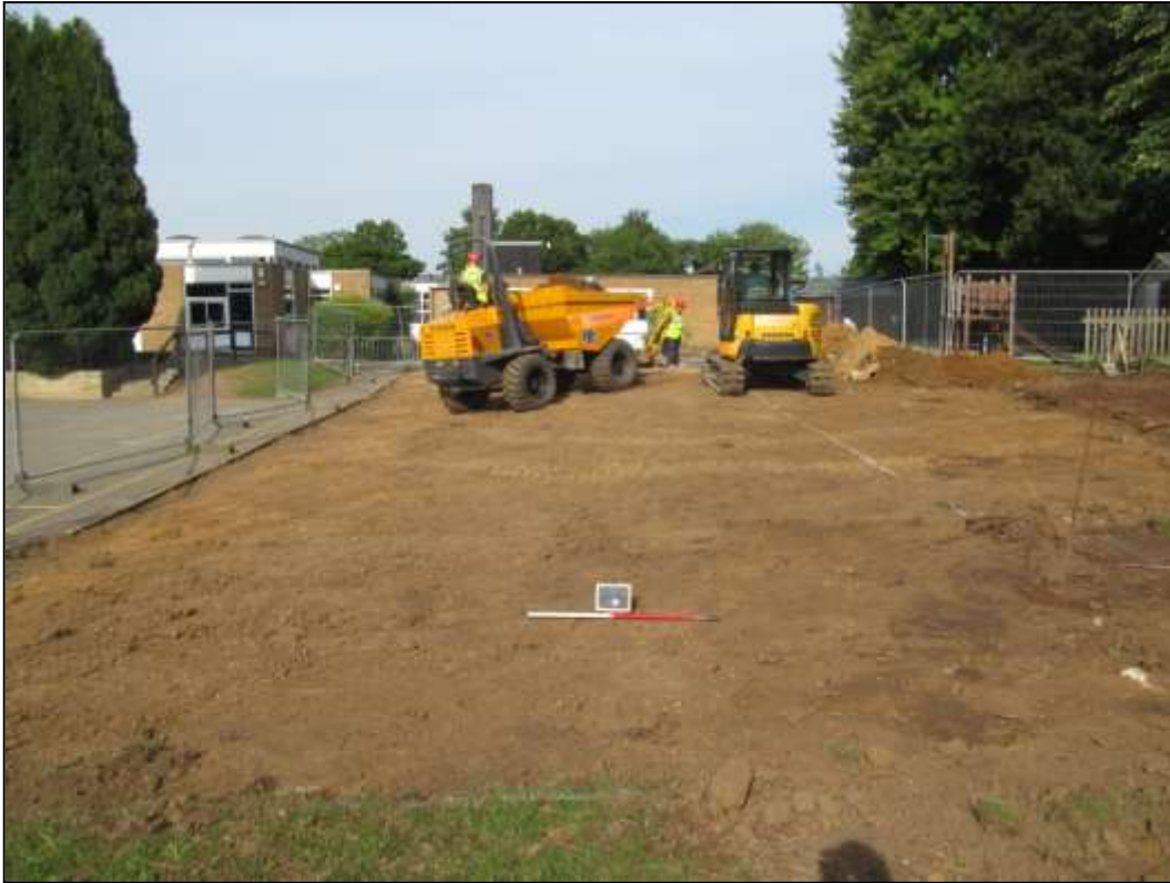
Plate 1: Site after topsoil strip, looking west.
