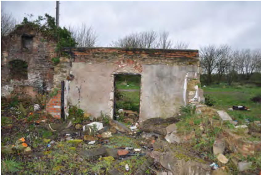
Plate 7: Surviving west end of north extension (Wall 256)
