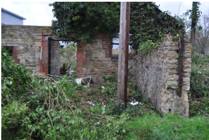
Plate 6: Surviving west gable end (Wall 824)
