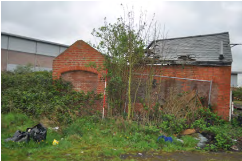
Plate 8: Building between east to west orientated building and Priory public house
