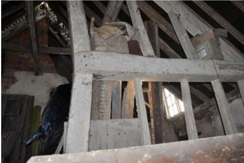
Plate 18: Truss in cheeseroom loft
