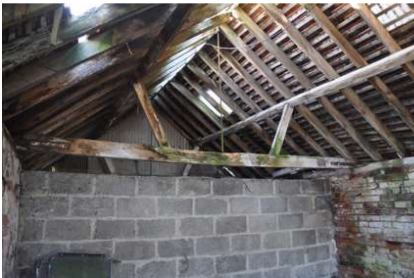
Plate 22: Milk Shed truss
