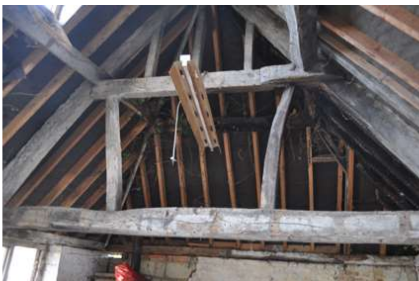
Plate 14: Truss in cheeseroom annex G8
