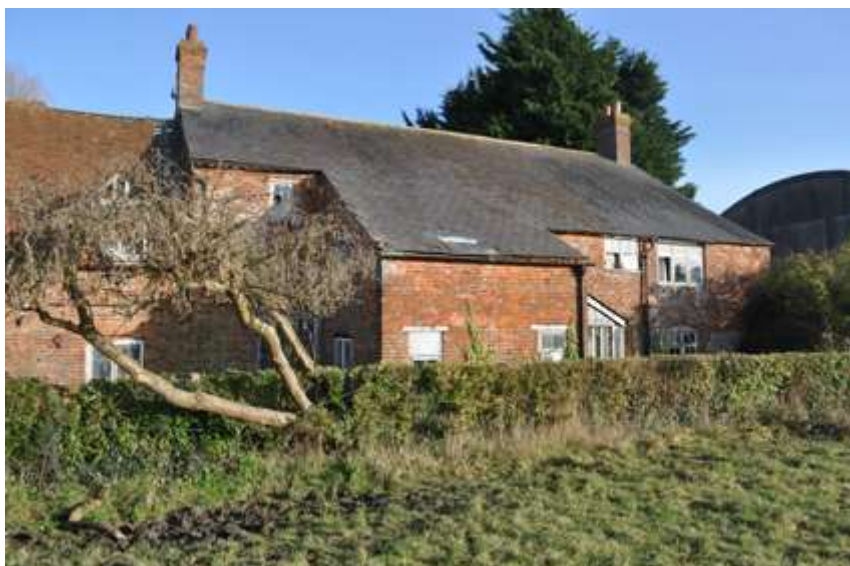
Plate 4: Rear façade of Farmhouse
