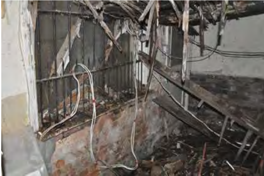
Plate 8: Room G2 north wall
