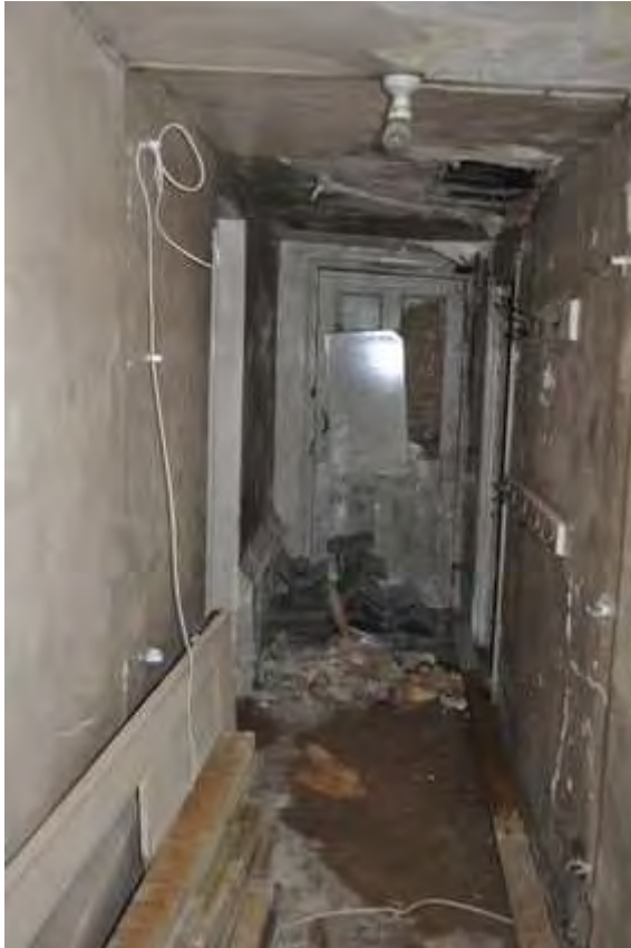
Plate 6: Passage G1 looking north
