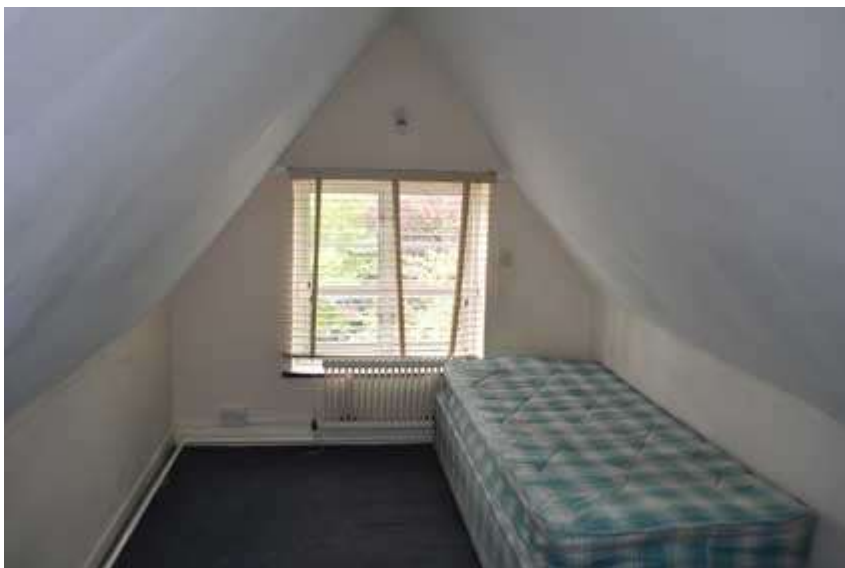
Plate 9 Gable interior A3
