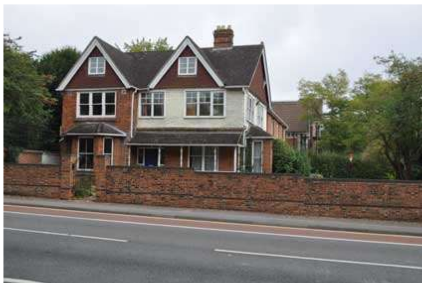
Plate 1 West and south façades
