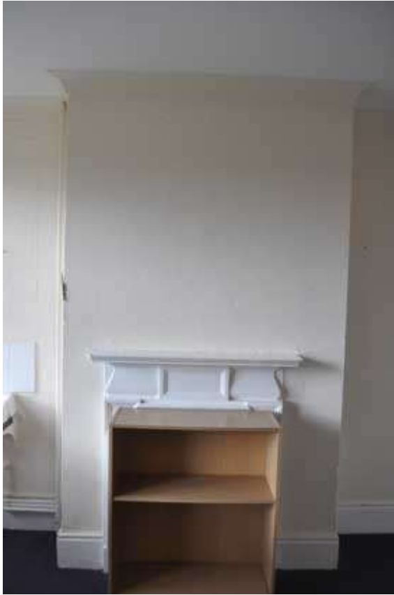
Plate 8 Chimney breast in F5
