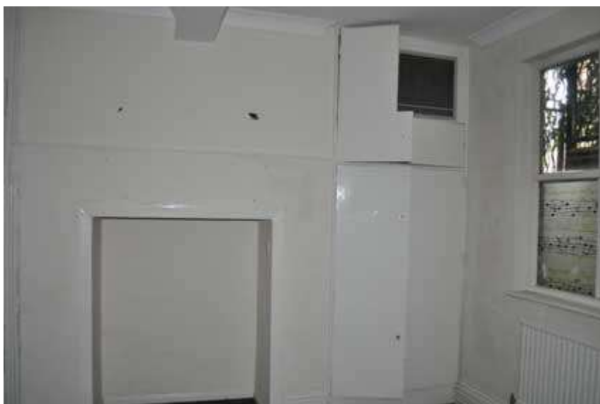
Plate 4 Fireplace in former kitchen (G5)
