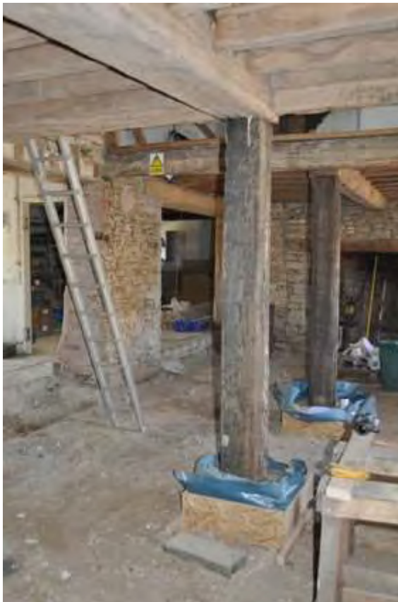
Plate 8: Timber posts and ceiling beams in stone building
