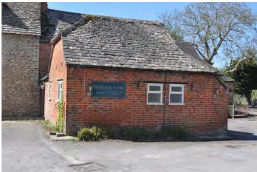
Plate 4: Front elevation of additional brick extension
