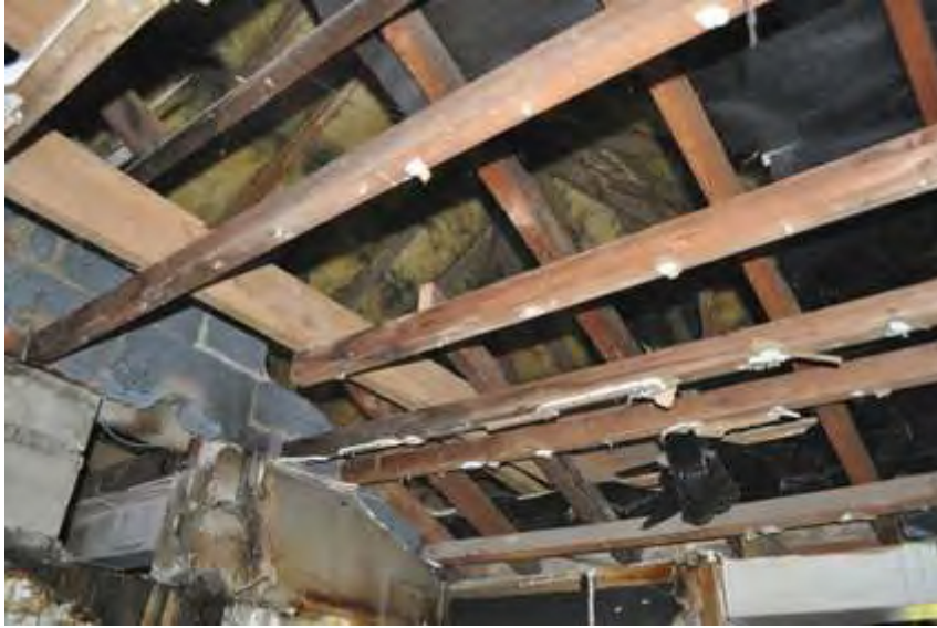
Plate 12: Exposed roof truss in kitchen
