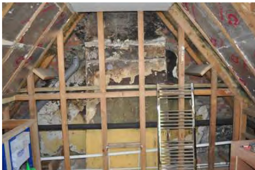
Plate 19: Chimney breast in bedroom
