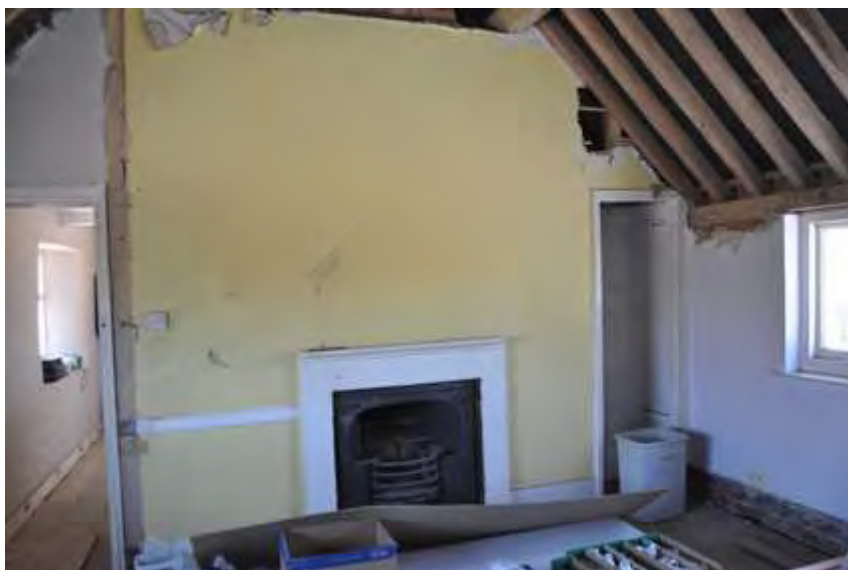
Plate 16: Fireplace in bedroom 1
