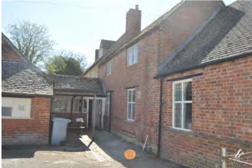
Plate 3: Front elevation of the brick extension
