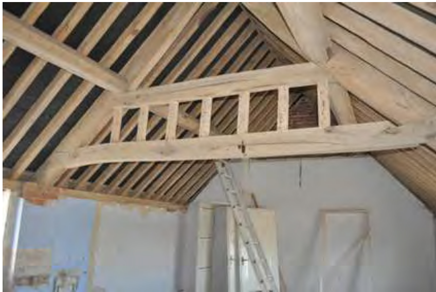
Plate 15: Timber truss in loft
