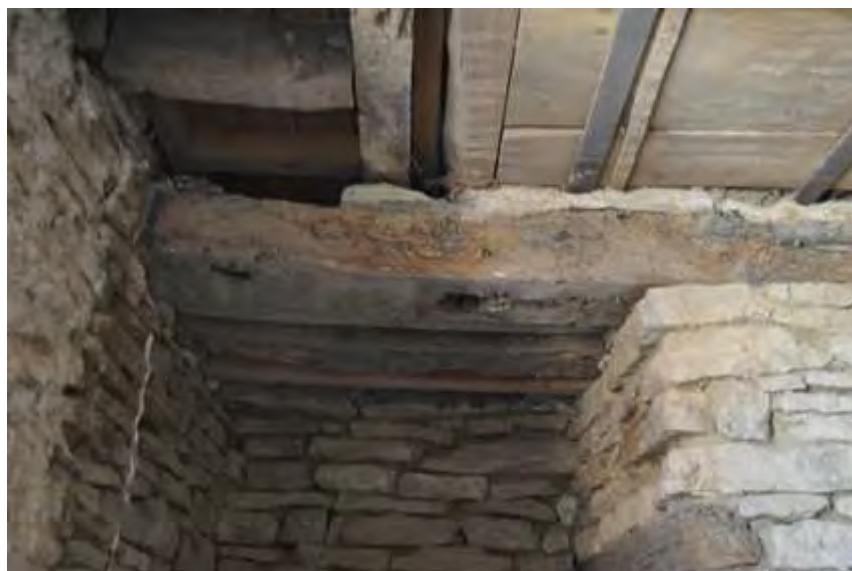
Plate 6: Timber beams at side of fireplace
