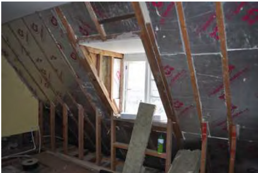
Plate 18: Roof truss and dormer window
