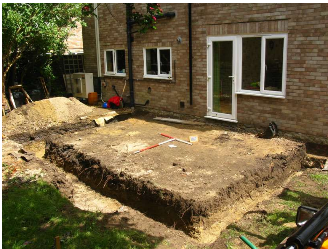
Plate 1: General overview of foundation trench, looking northeast
