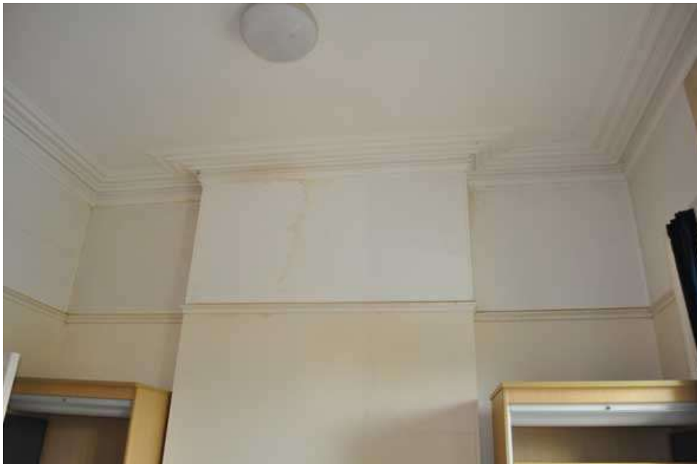
Plate 24: Chimneybreast and moulding, bedroom
