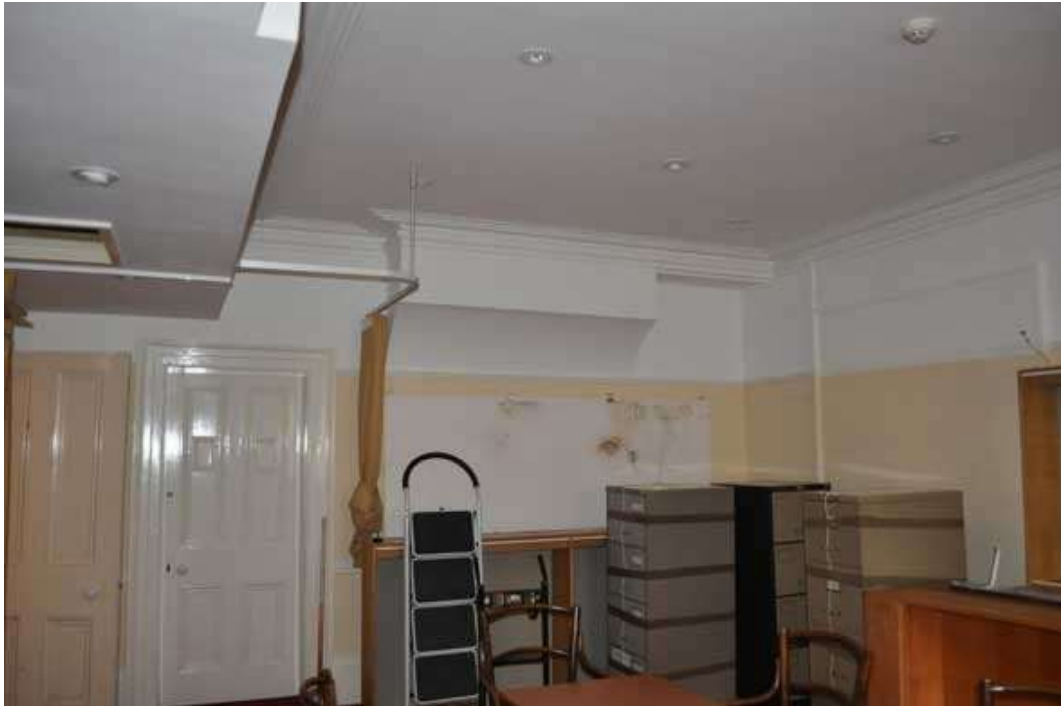
Plate 29: Northwest room, first floor
