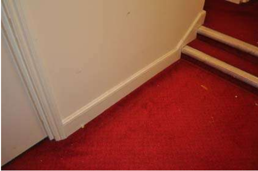
Plate 23: Replaced skirting, L-shaped passage
