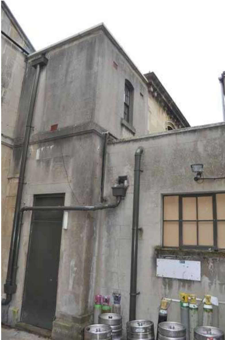
Plate 4: New construction on the north façade
