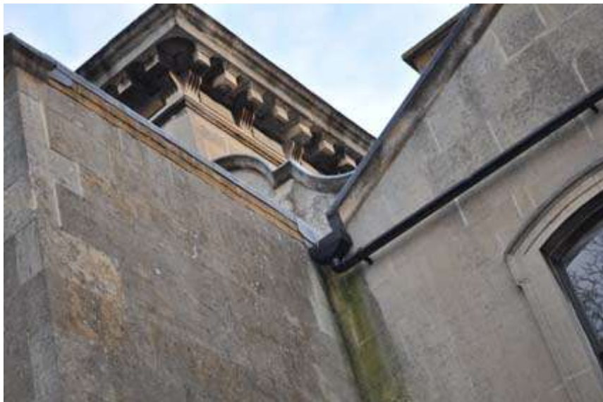
Plate 6: Partial gable end associated with stair access to second floor of tower
