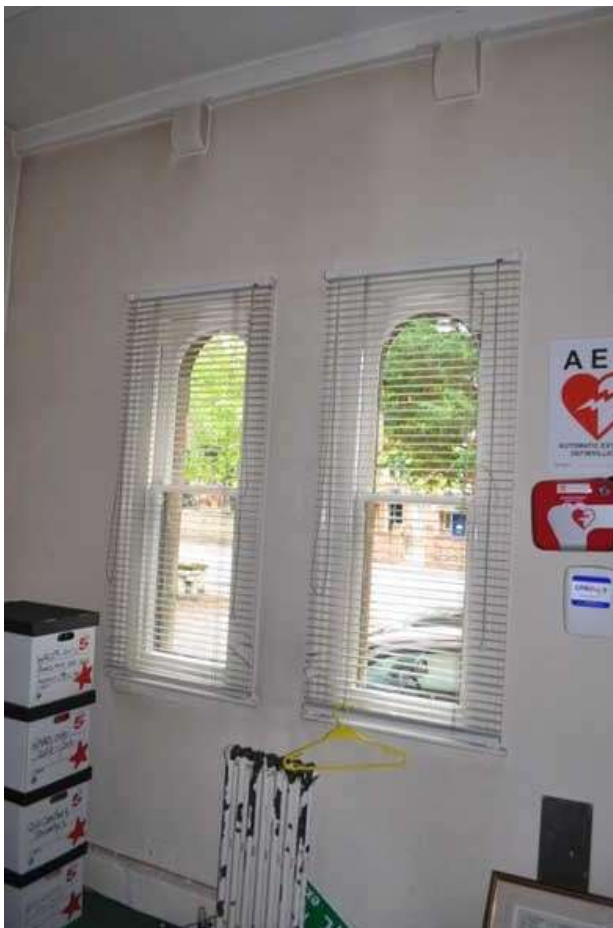
Plate 19: Reinstated windows in the northeast wing
