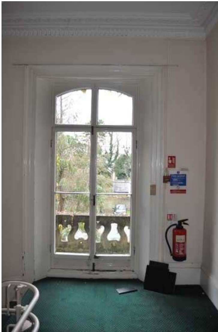
Plate 21: Balcony door, landing
