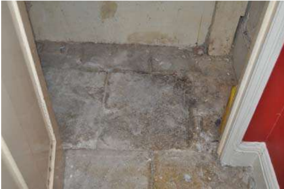
Plate 18: Flagstone flooring, scullery
