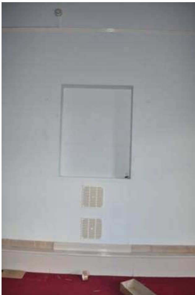
Plate 33: Temple Room original door
