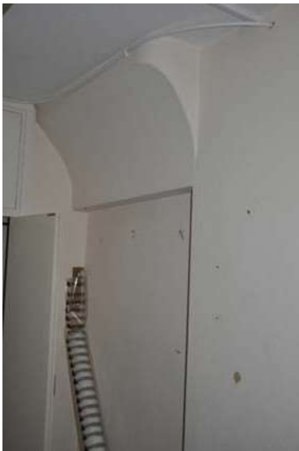
Plate 20: Chimney breast, northeast wing
