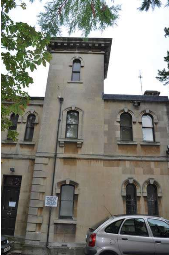
Plate 8: Tower, east façade
