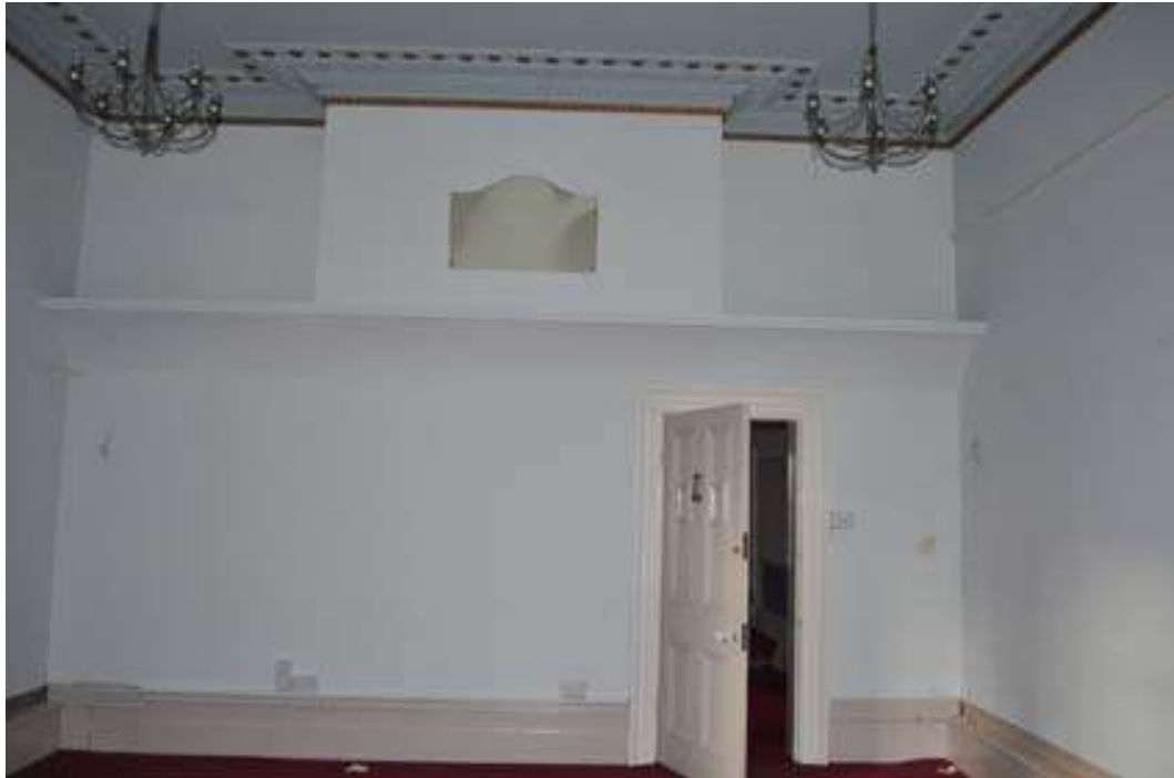
Plate 32: Temple Room, remains of chimneybreast
