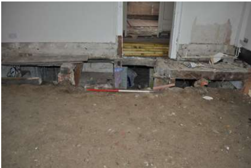
Plate 14: Edge of cellar as seen from room G2
