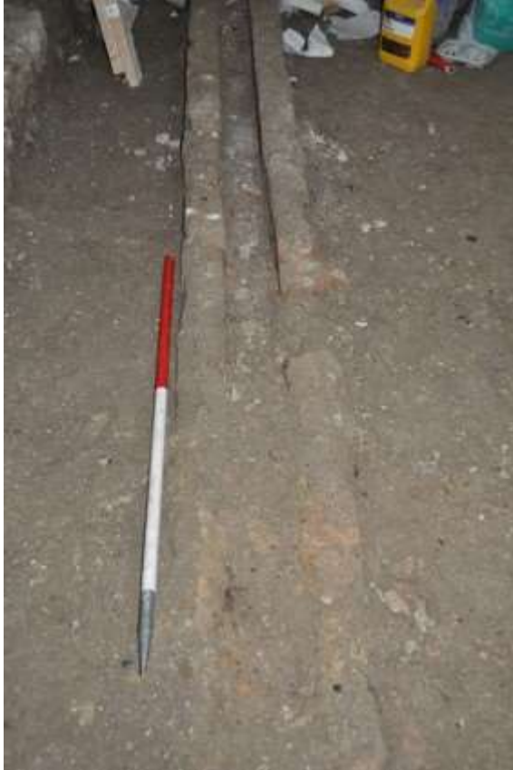
Plate 15: Brick channel in room G2
