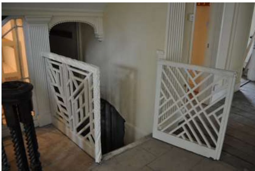
Plate 9: Cellar entrance G1
