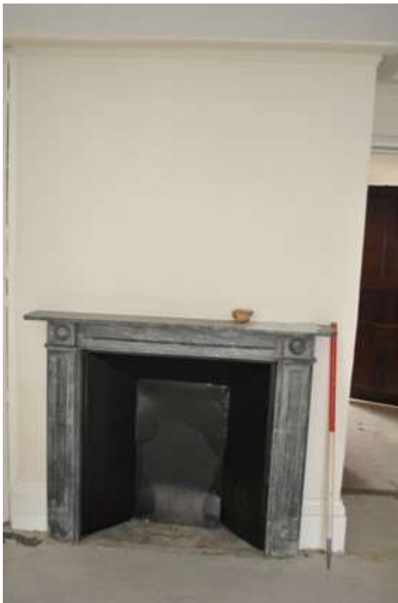
Plate 11: Chimneybreast in room G2
