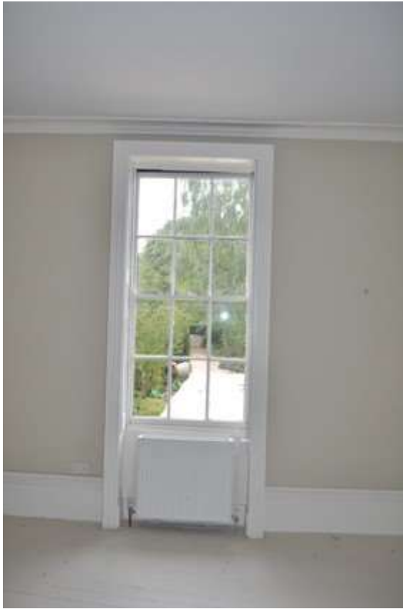
Plate 20: Window room F3
