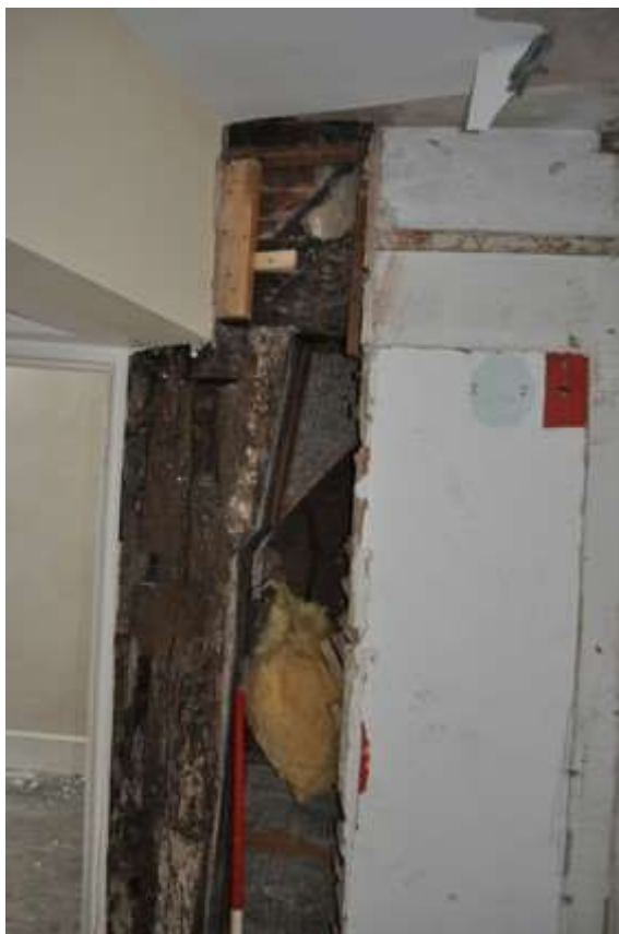
Plate 25: Kerb principal truss in F2a
