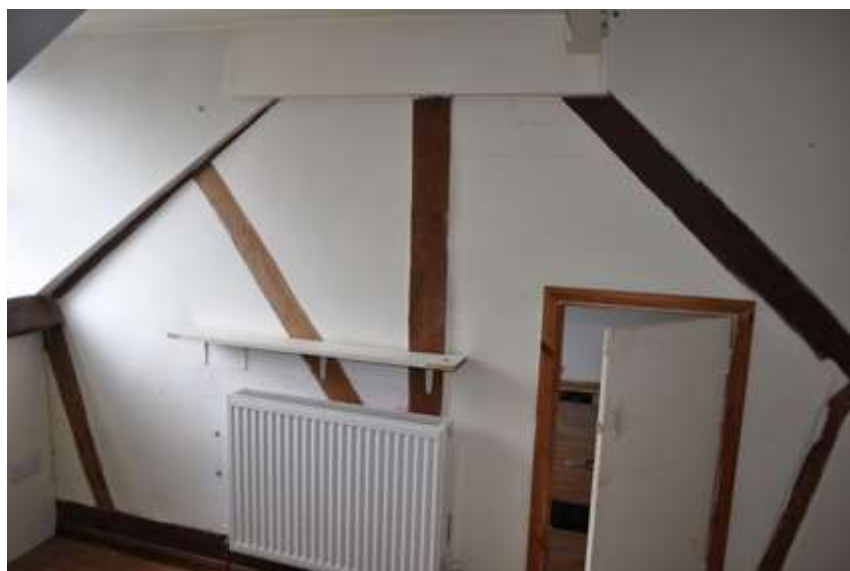
Plate 26: Truss in rear of second floor
