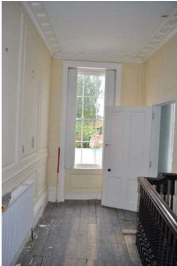
Plate 17: Landing F1 looking south
