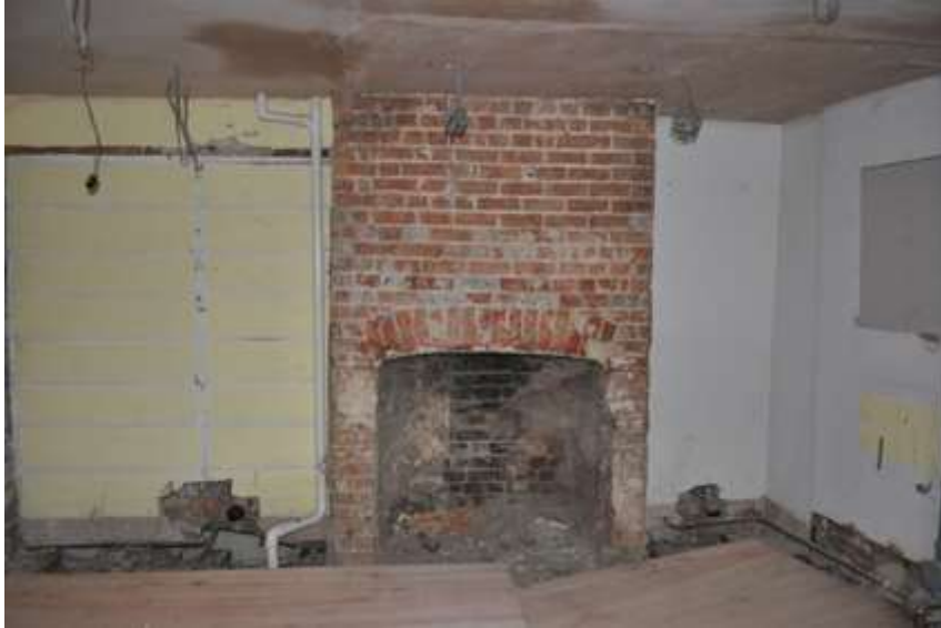
Plate 10: Stripped out room G4 with uncovered chimneybreast
