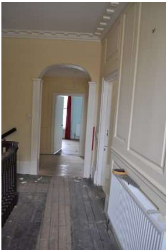
Plate 18: Landing F1 looking north
