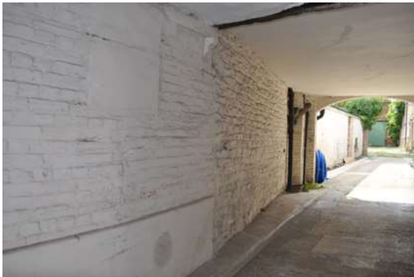
Plate 6: Cart way with remains of timber framing
