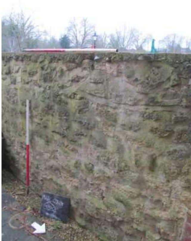
Plate 3: Boundary wall 1000, showing part of area dismantled
