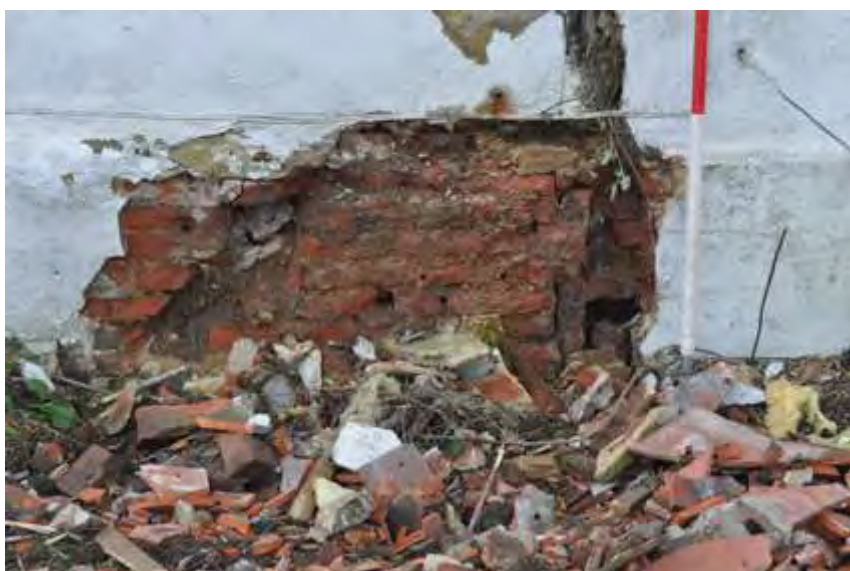
Plate 9: Plinth on north façade (wall 2/12)
