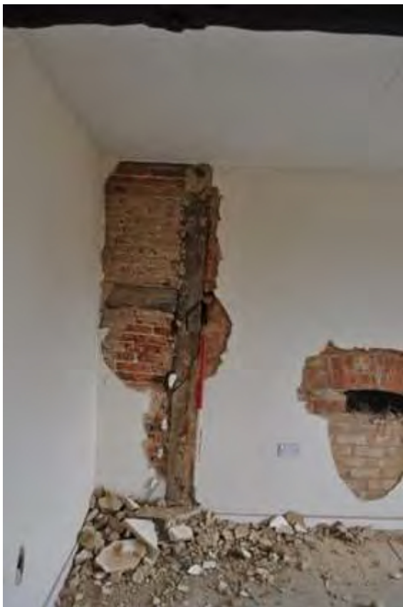
Plate 22: Timber framing F7
