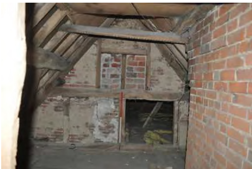
Plate 28: Attic A trusses
