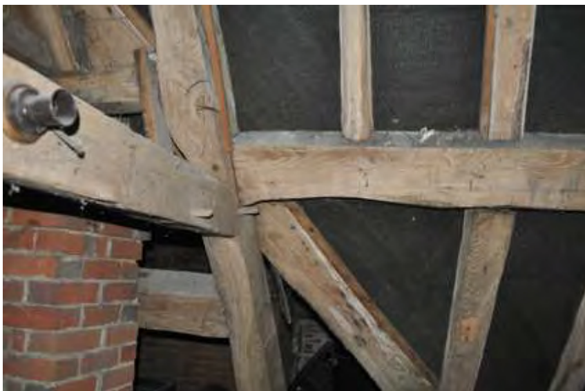
Plate 25: Attic A trusses
