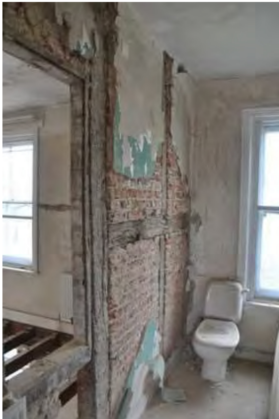
Plate 20: Timber framing F5
