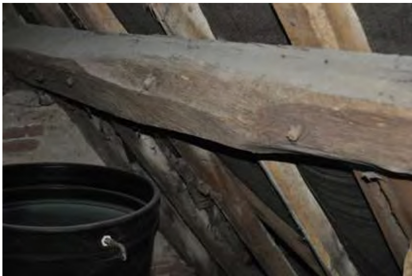
Plate 30: Attic A perlins
