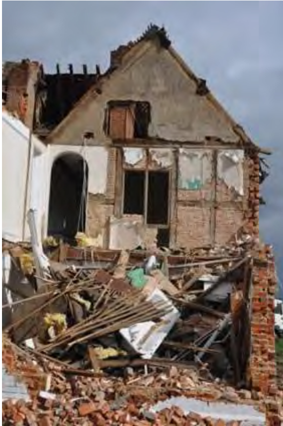
Plate 21: Timber framing F1a and F5
