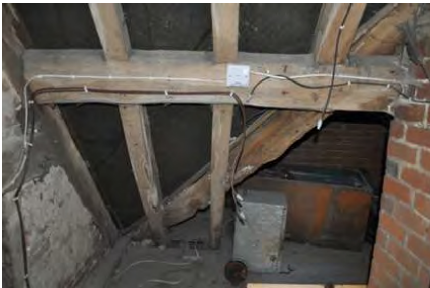
Plate 27: Attic A perlins
