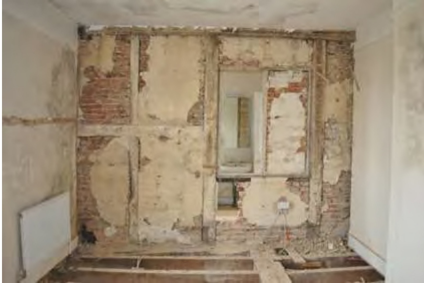
Plate 18: South wall F3
