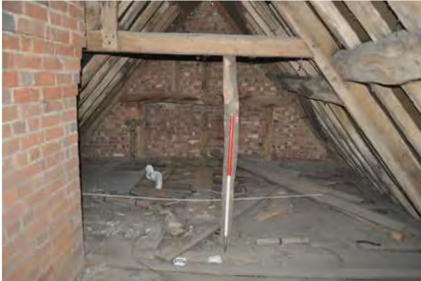
Plate 23: Attic A trusses
