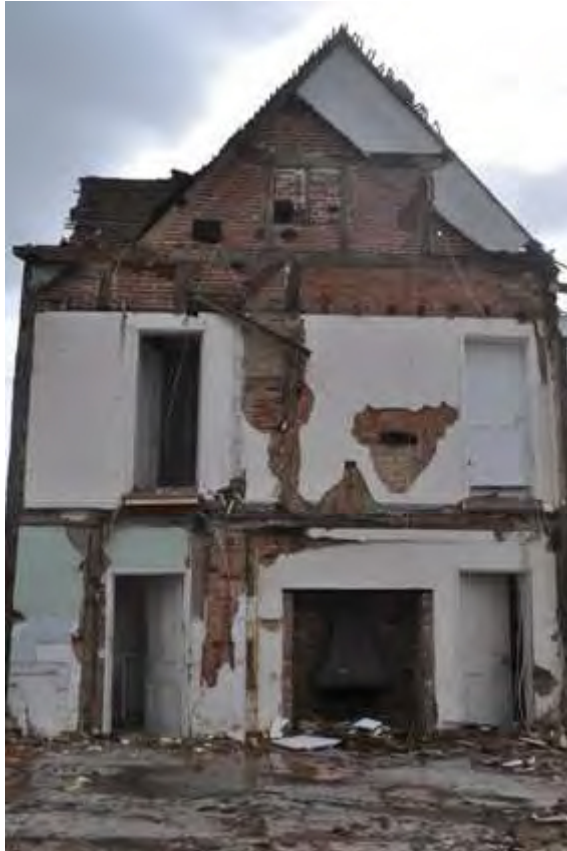
Plate 6: Former west gable
