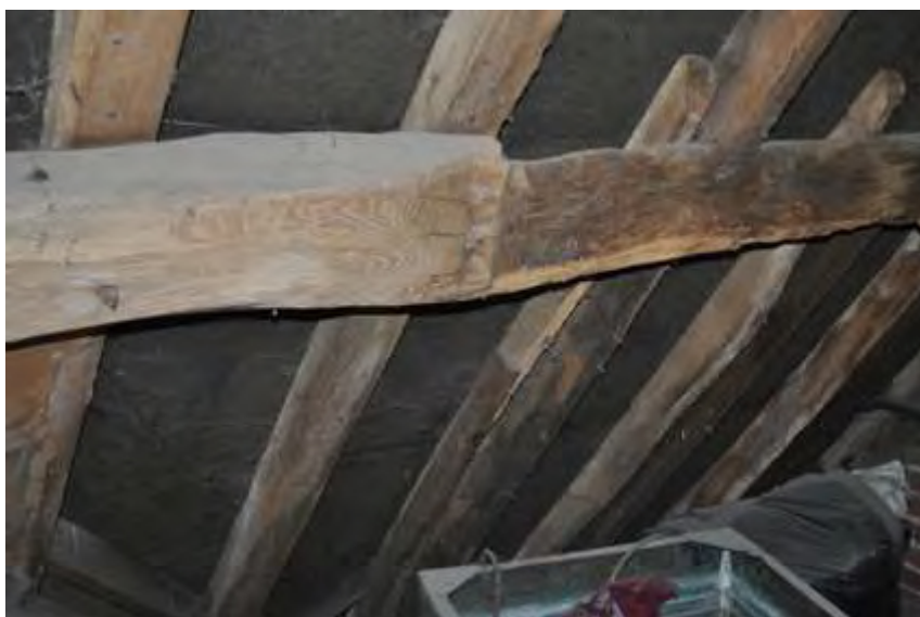
Plate 31: Attic A perlins
