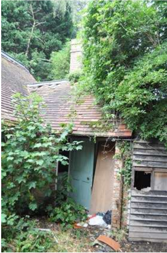
Plate 3 South elevation east end porch
