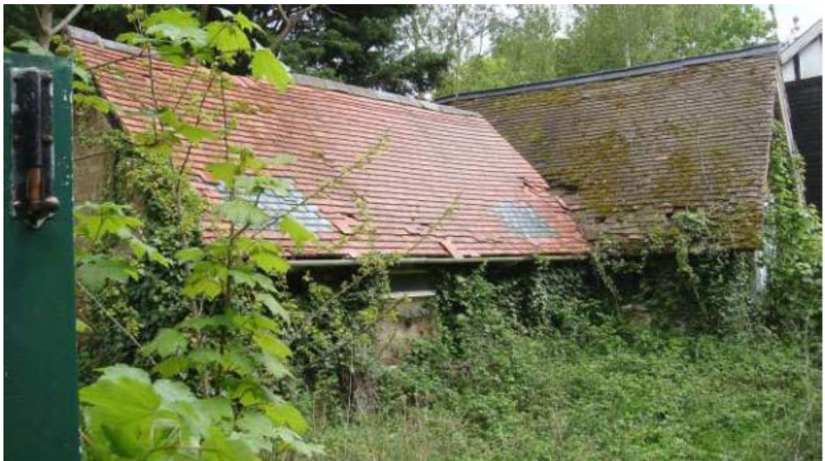
Plate 1 South elevation west end
