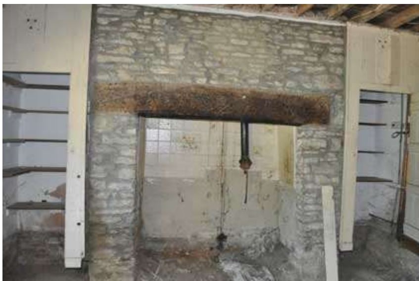
Plate 6 Cupboard fittings either side of fireplace (G6)
