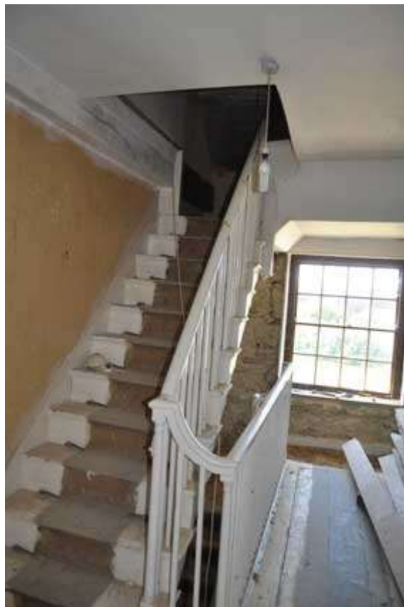
Plate 8 Stairs on landing (F1)
