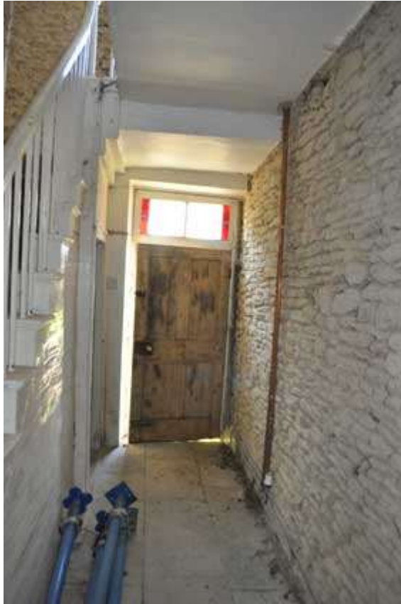
Plate 3 Internal view of front door
