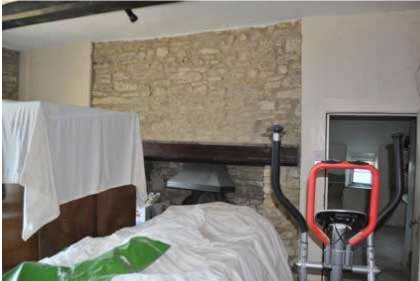
Plate 4 Panelled cupboards either side of fireplace (G3)
