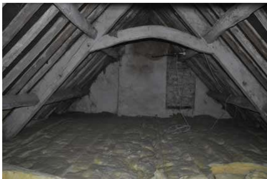
Plate 10 Bowed cross beam (A5)
