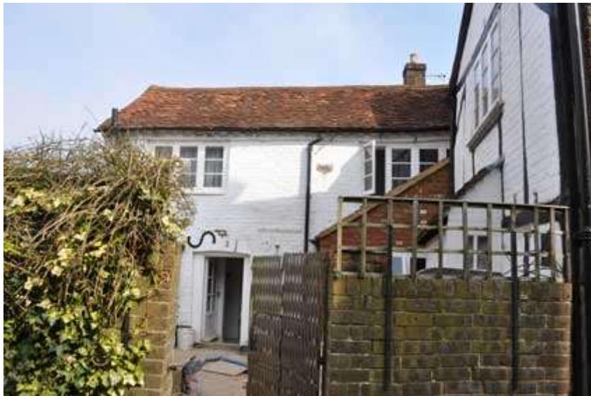
Plate 3 Southwest elevation of rear wing
