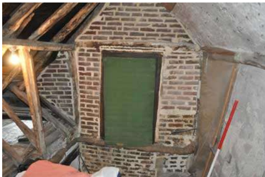
Plate 11 Internal part of rear central gable, attic
