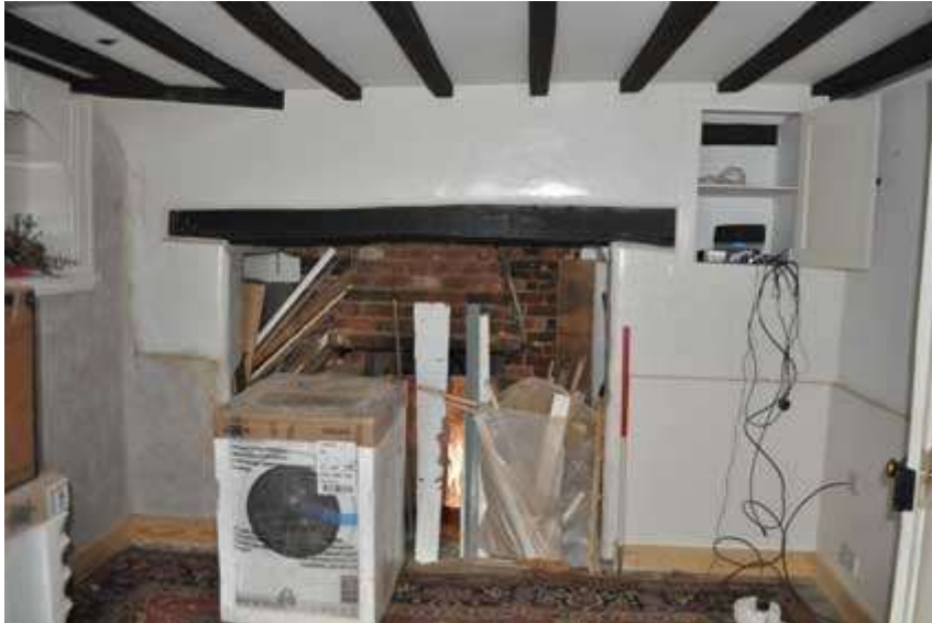
Plate 6 Ground floor southeast room (G2), fireplace
