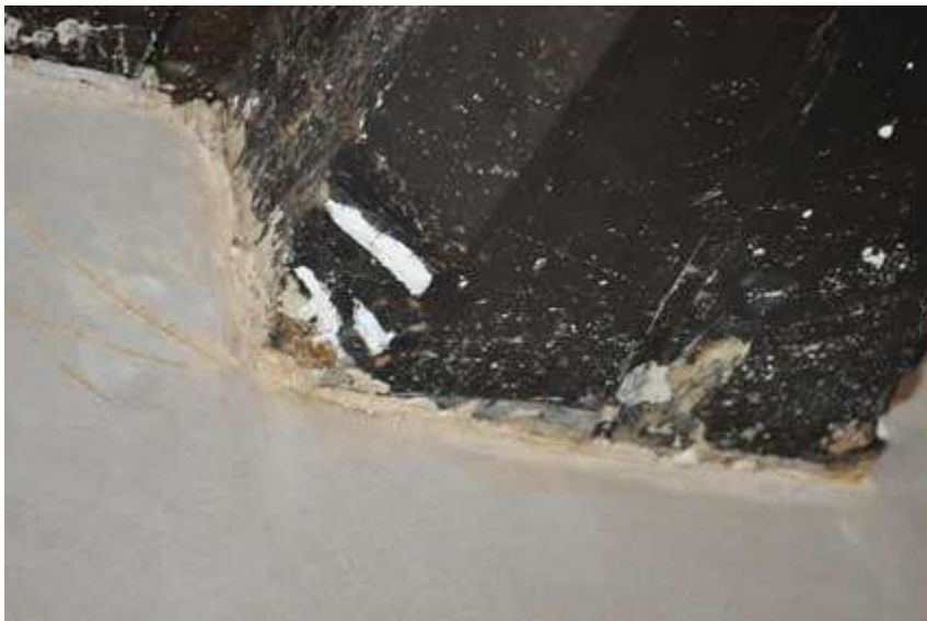
Plate 7 Chamfer and stop at the end of the beam
