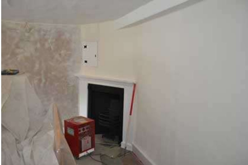
Plate 9 Fireplace southeast room (F2), first floor
