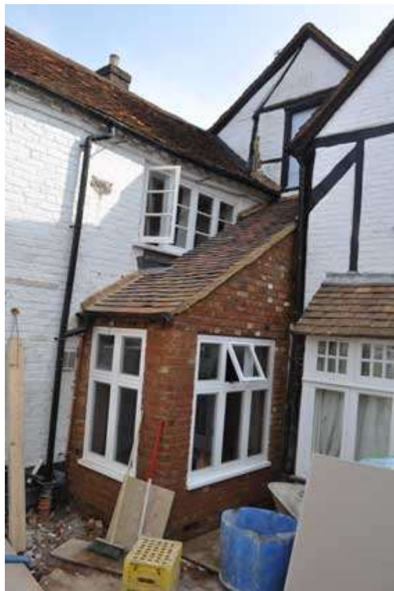
Plate 4 Rear or northwest façade
