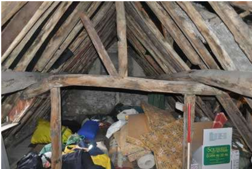
Plate 10 Central truss, attic
