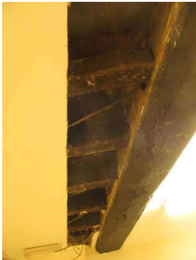
Plate 4 Chamfered beam in C3
