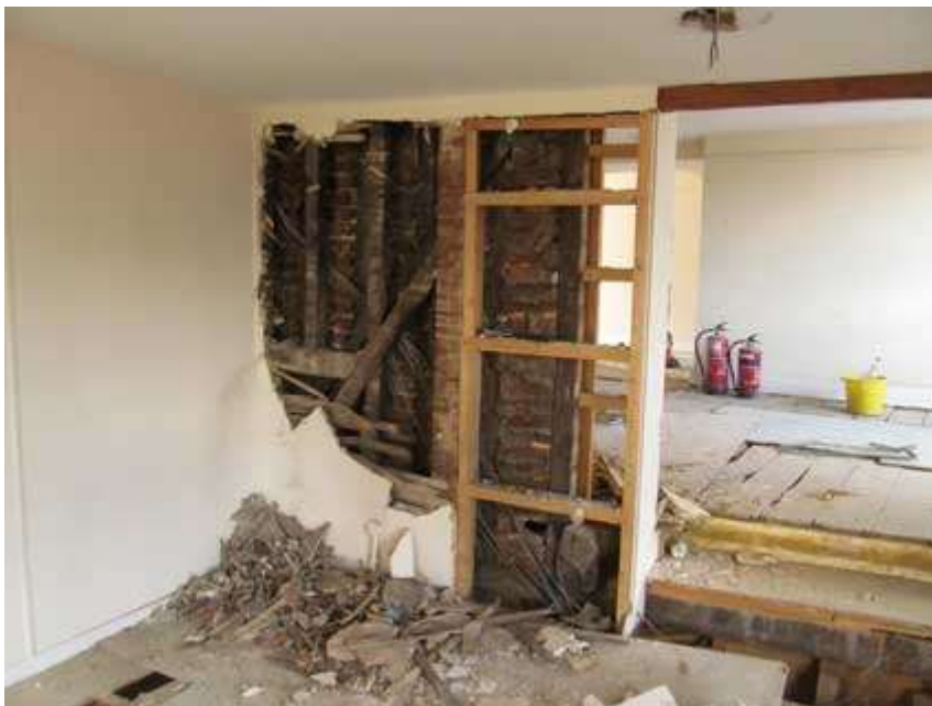
Plate 6 Wall between S1 and S2 from the east
