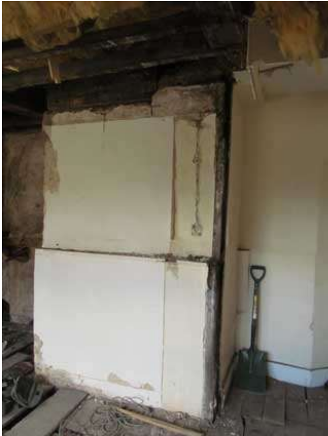
Plate 9 Chimneybreast in south wall of T3
