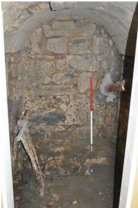
Plate 3 Stone wall and vault under the pavement
