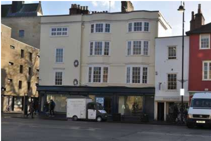
Plate 1 Broad Street façade
