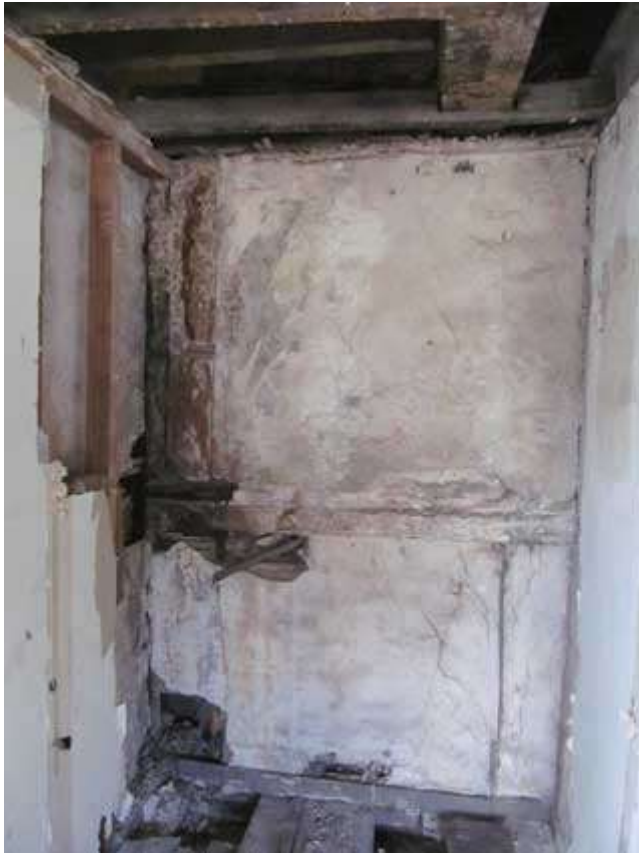
Plate 7 Timber framing in south of room T3
