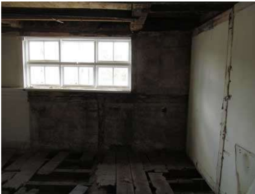
Plate 8 Timber framing in wall on north side of T3
