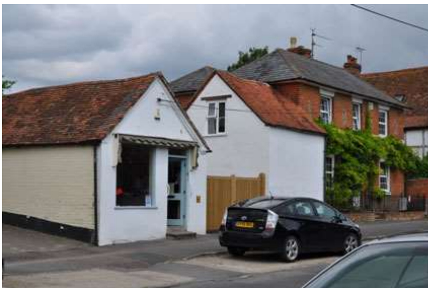
Plate 2 Front façade of southern linear shaped building and parts of east façade.
