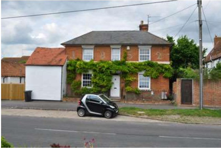
Plate 1 Front façade of Wilcote House
