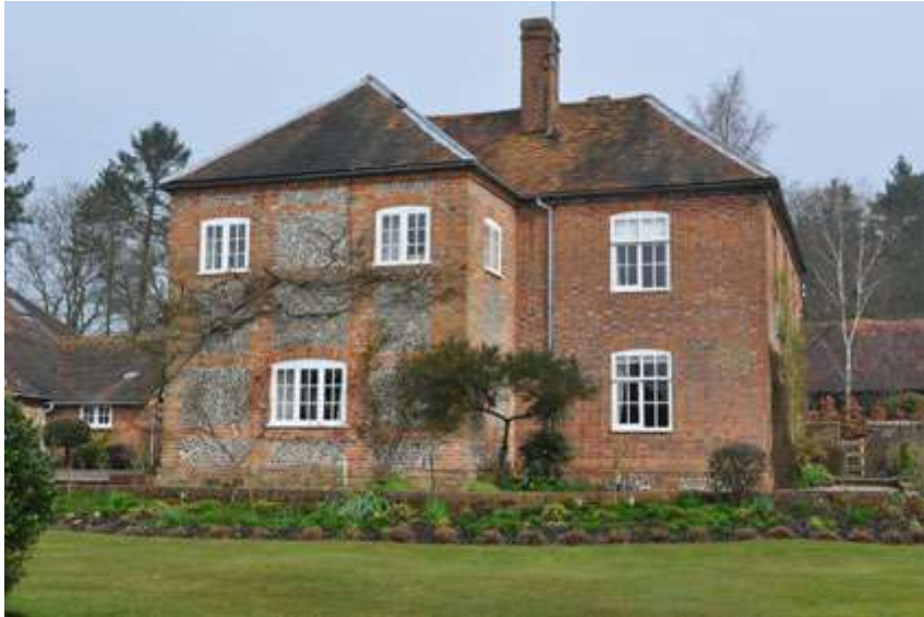
Plate 2 South façade details
