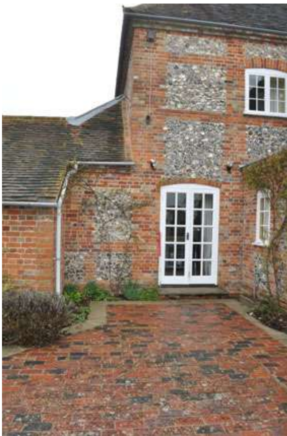
Plate 3 South façade details (butt joint)
