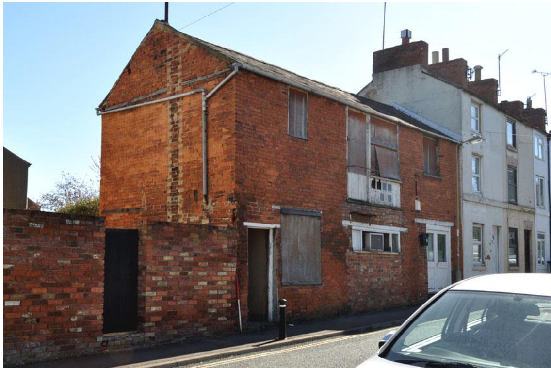
Plate 2. View from the west corner
