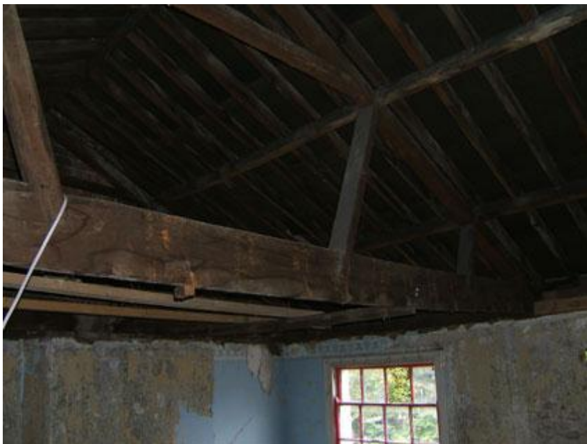
Plate 13: Truss arrangements
