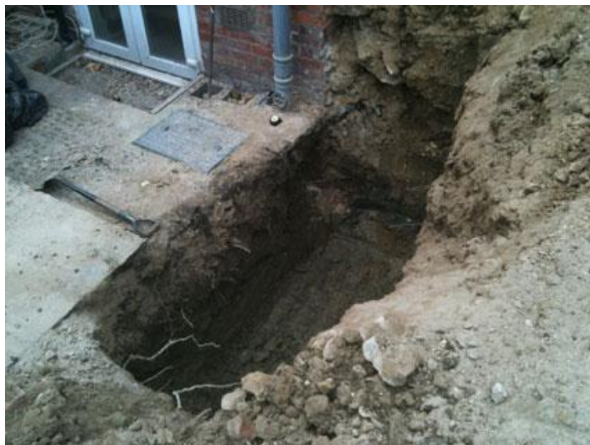
Plate 18: Foundation trench on boundary with no. 63 (possible stone boundary wall)
