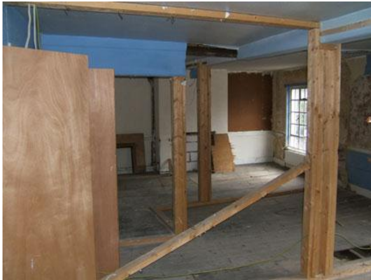
Plate 10: Views of the first floor
