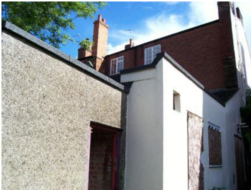
Plate 4: Southwest elevation from rear
