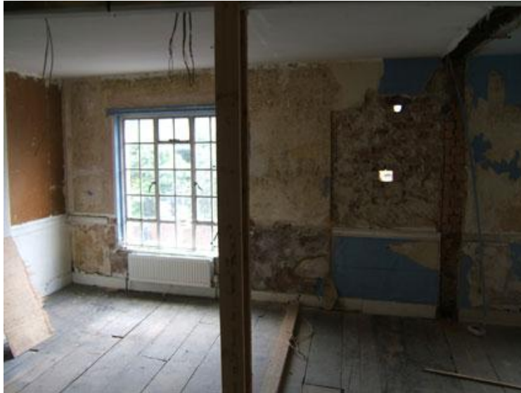
Plate 9: Views of the first floor
