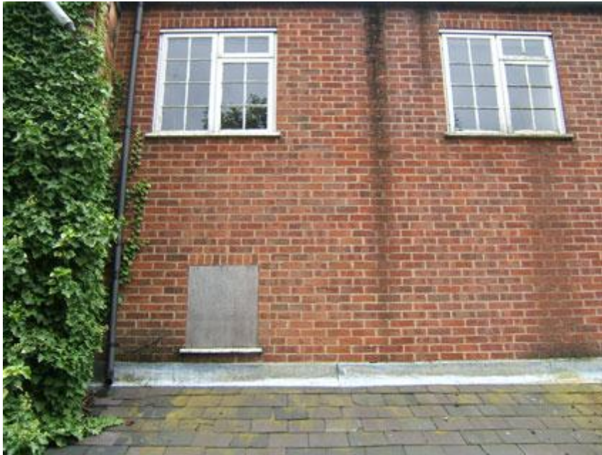
Plate 5: Modern rear wall, northwest elevation
