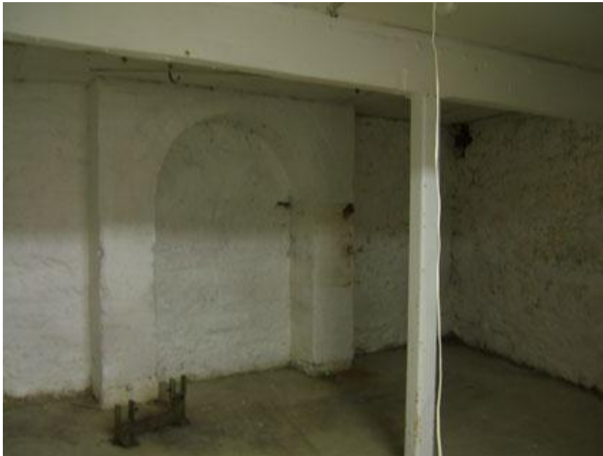
Plate 17: Base of northeast chimneybreast in cellar
