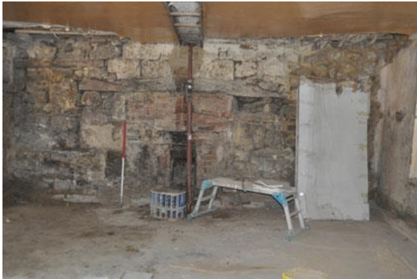
Plate 6. Uncovered fireplace east unit ground floor
