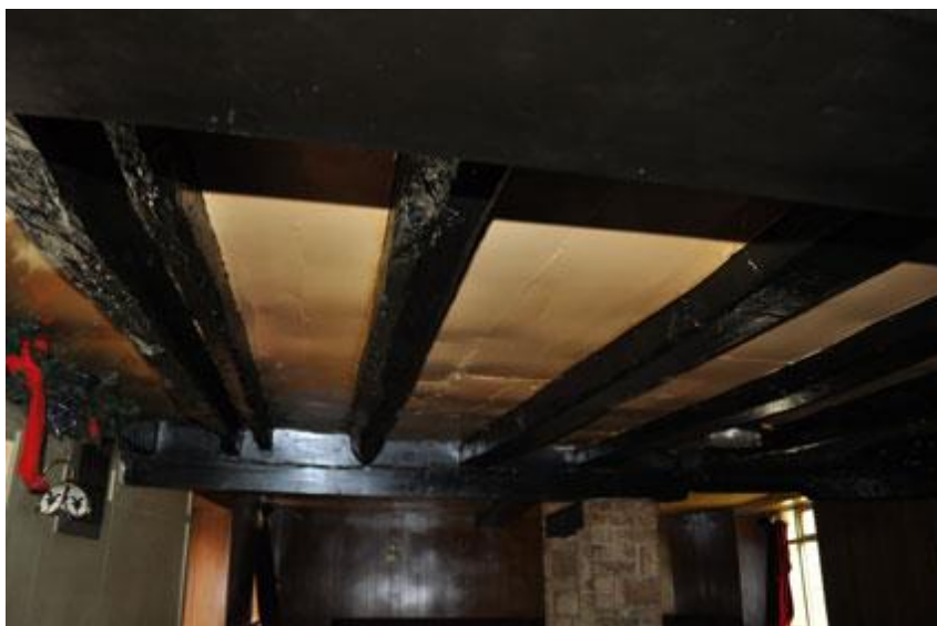
Plate 4. Timbers in central unit ground floor
