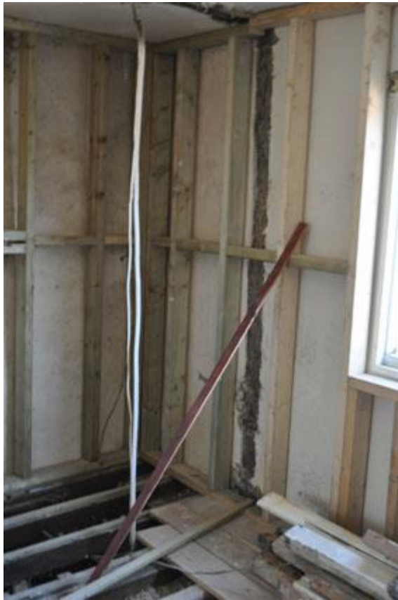
Plate 8. External timber framing seen below framing for dry walling
