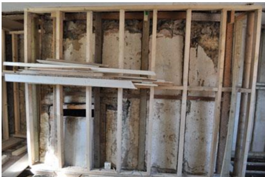
Plate 7. Uncovered fireplace and chimney breast, west unit first floor
