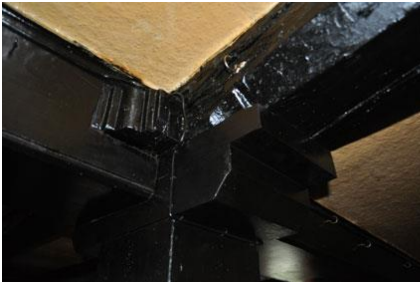
Plate 3. Stop on chamfered beam west unit ground floor
