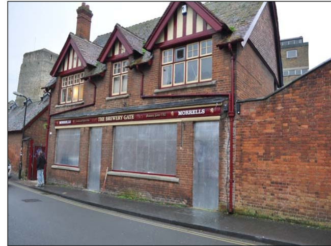
Plate 2. Brewery Gate, north facade
