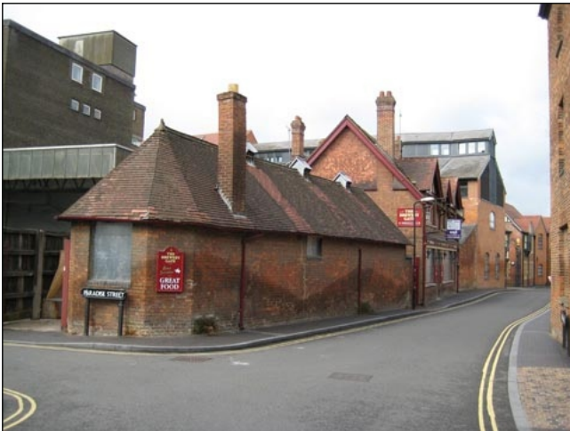
Plate 3. Brewery Gate, north and east facades
