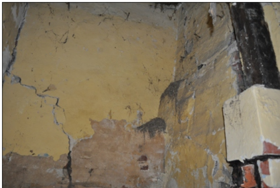
Plate 3. Remains of floor and step lines, indication of earlier stairwell.
