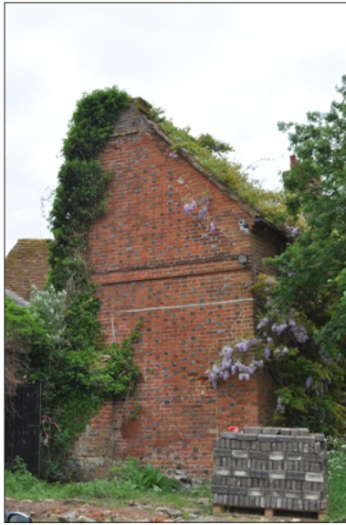
Plate 1. Gable End, west.
