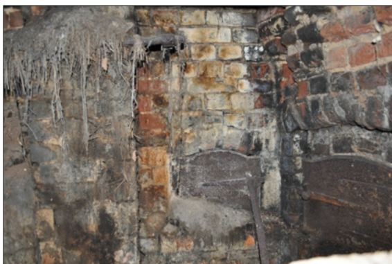
Plate 5. Oven doors inside fireplace.
