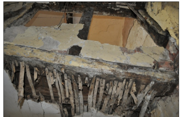
Plate 4. Wall through which staircase would lead.
