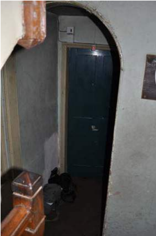
Plate 37. Archway to be lost adjacent to stairwell
