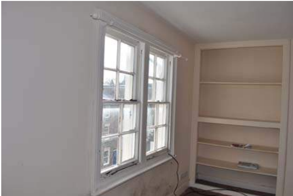
Plate 32. Second floor mullioned window, Stert unit
