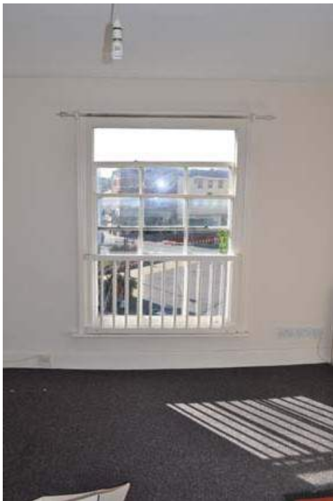
Plate 31. Second floor, sash window Market Square unit
