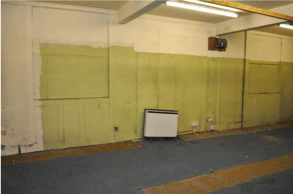
Plate 10. Ground floor, apparent wooden frame behind the Stert Street brick facade
