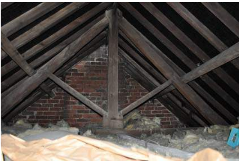
Plate 36. Attic Stert Street unit
