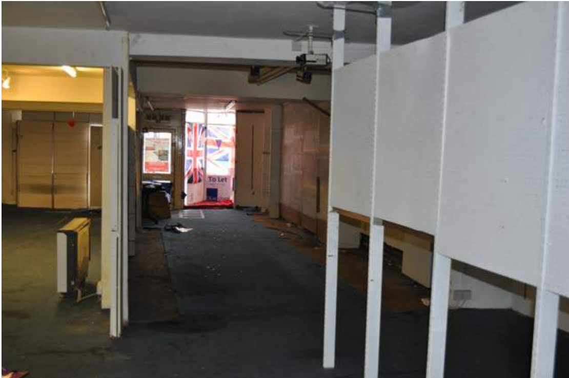
Plate 9. General view of gutted ground floor
