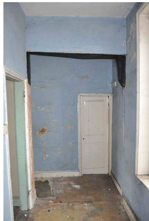
Plate 18. Area where timber frame has been partially removed
