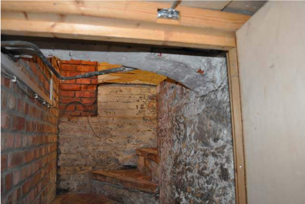
Plate 23. Stairwell into cellar
