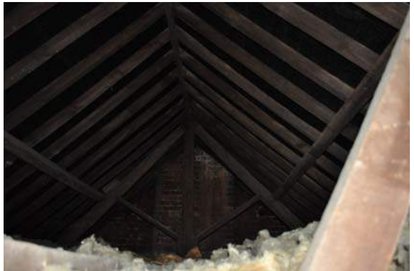
Plate 33. Attic Stert Street unit
