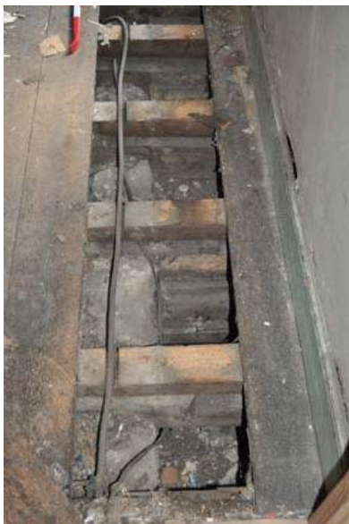
Plate 28. First floor, Market-Stert unit, Limestone rubble wall surviving
