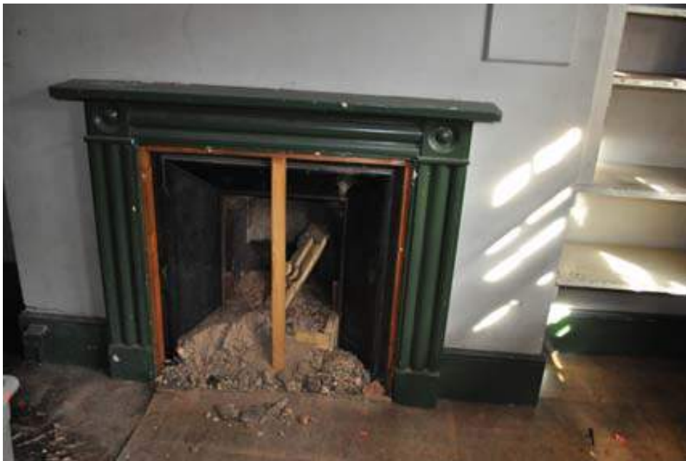
Plate 25. First floor, Stert unit, north fireplace
