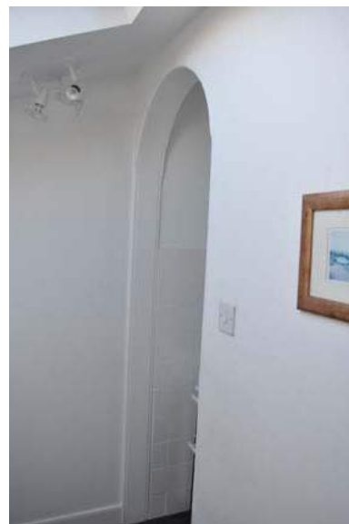
Plate 29. Second floor, Market Square unit, round-headed arch
