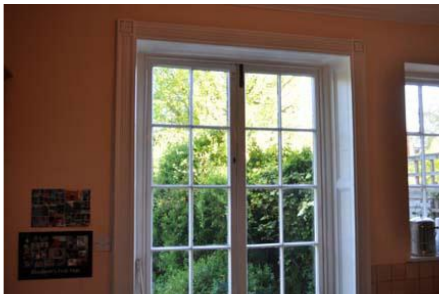
Plate 4. Patio door in kitchen
