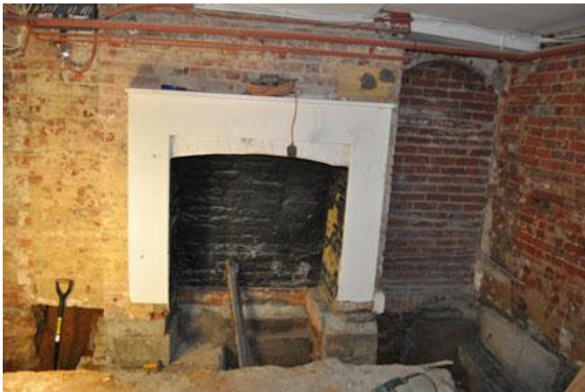
Plate 9. Fireplace in basement, with segmental arch alongside
