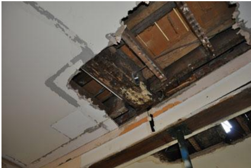
Plate 7. The large chamfered transverse timber beams
