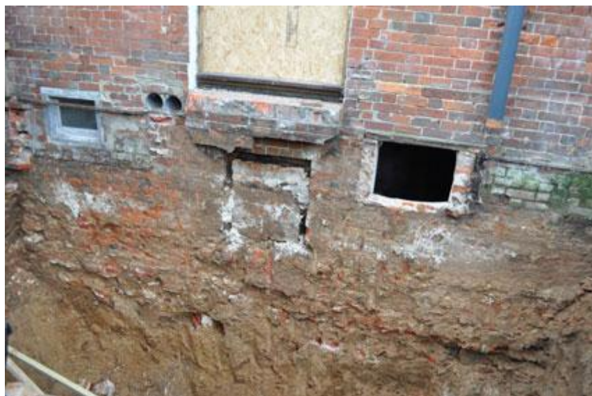
Plate 11. Features below the line of the patio northwest wall
