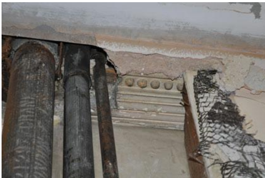
Plate 6. The remaining earlier ceiling plasterwork
