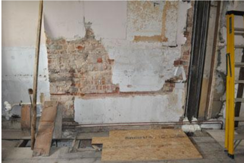
Plate 5. Part of the segmental arch in the kitchen chimneybreast
