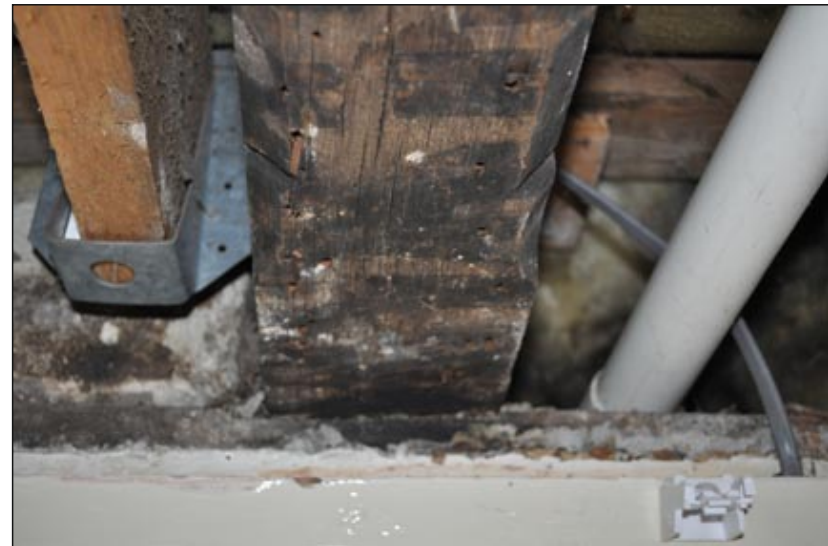
Plate 13. Hall ceiling details
