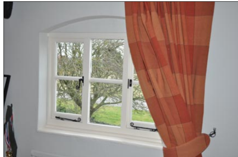
Plate 25. Bedroom, phase 6, north room west wing, window details
