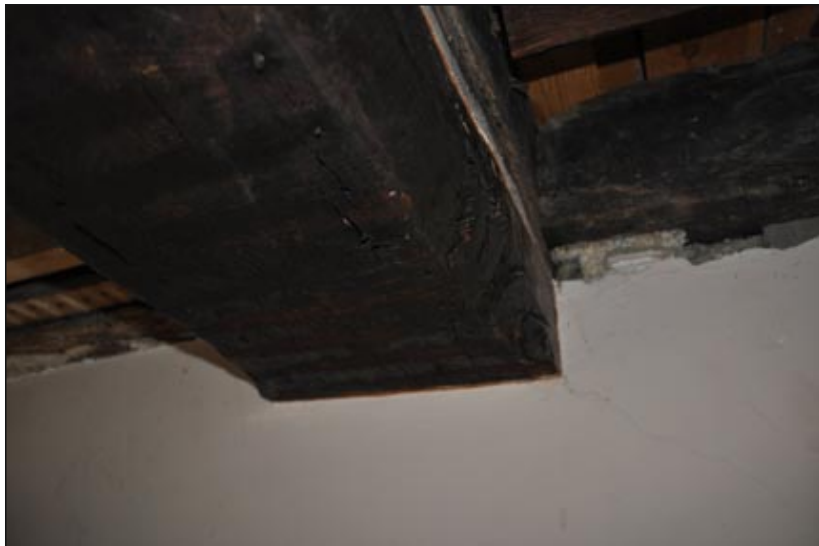
Plate 12. Hall ceiling details
