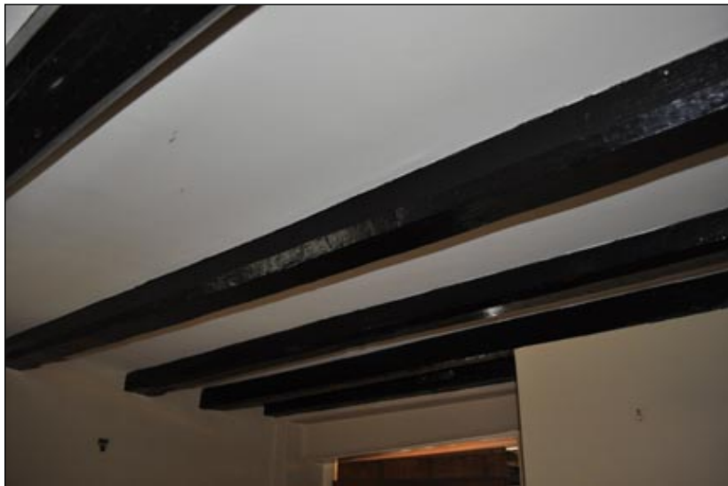
Plate 20. Living room, phase 4, ceiling details
