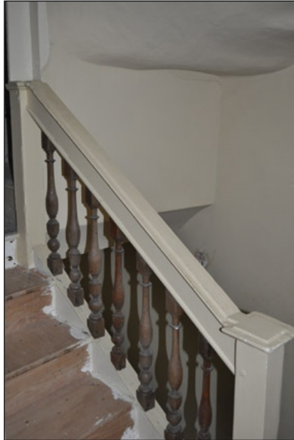
Plate 26. Stairs in stair tower
