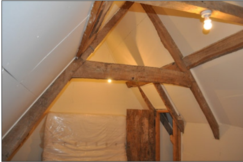
Plate 30. Trusses in garret
