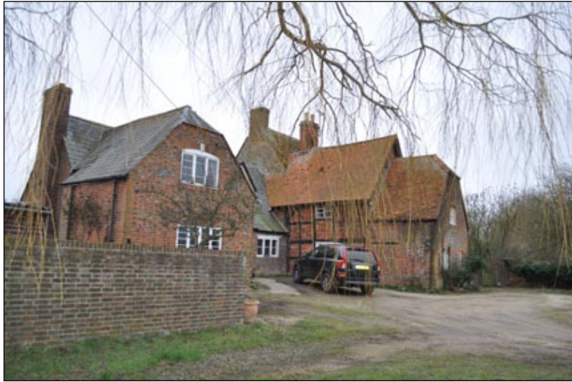
Plate 2. North elevations of Pound Farm
