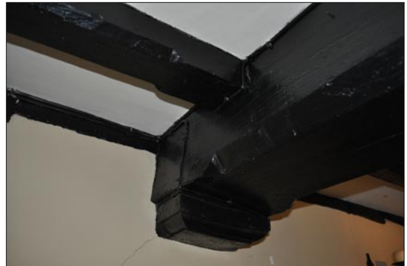
Plate 21. Living room, phase 4, ceiling details
