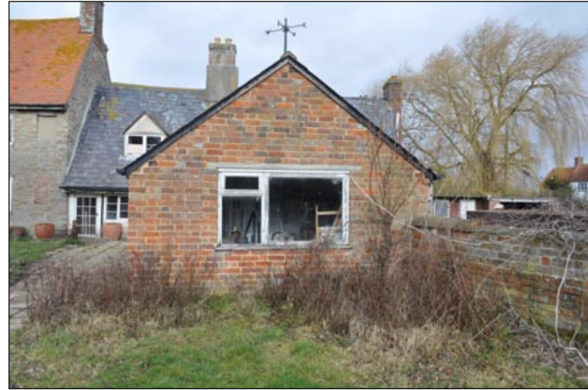
Plate 7. South elevation of Pound Farm out building
