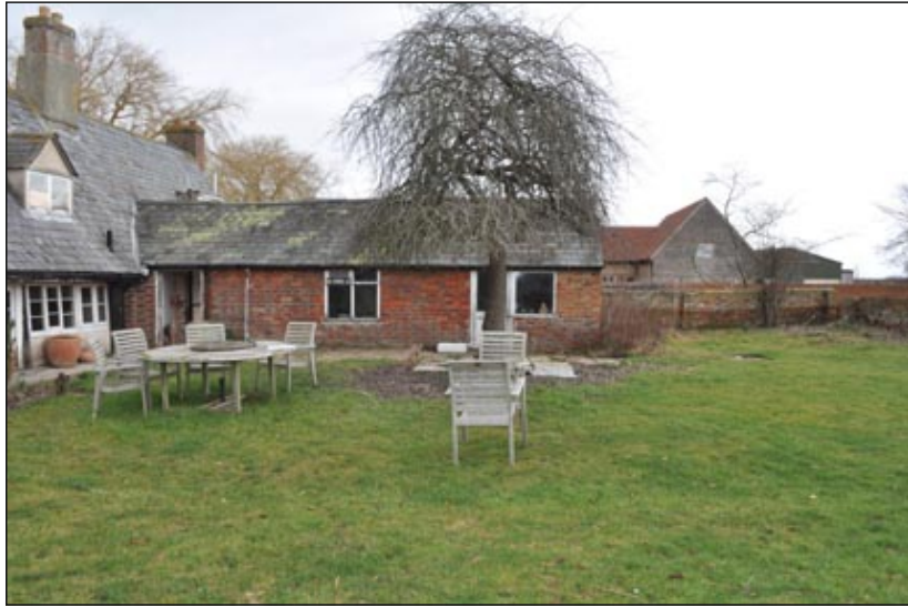
Plate 6. West elevation of Pound Farm out building
