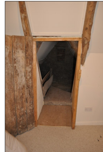
Plate 29. Upper part of stair tower
