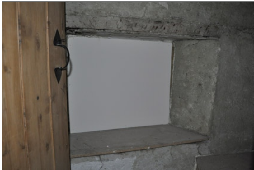
Plate 28. Blocked window, stair tower
