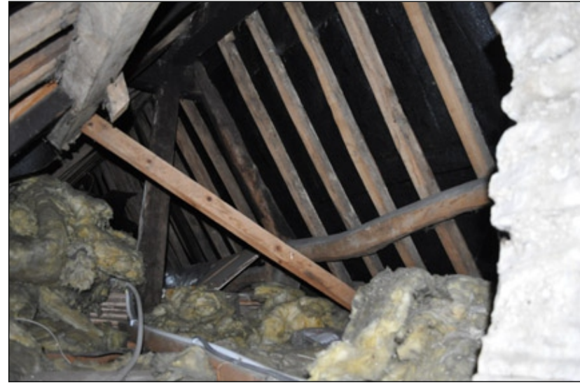
Plate 31. King stud in attic of central range
