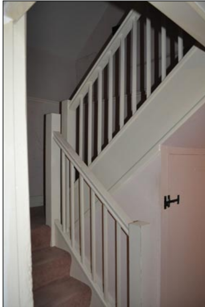
Plate 14. Hall, east stairs (modern)
