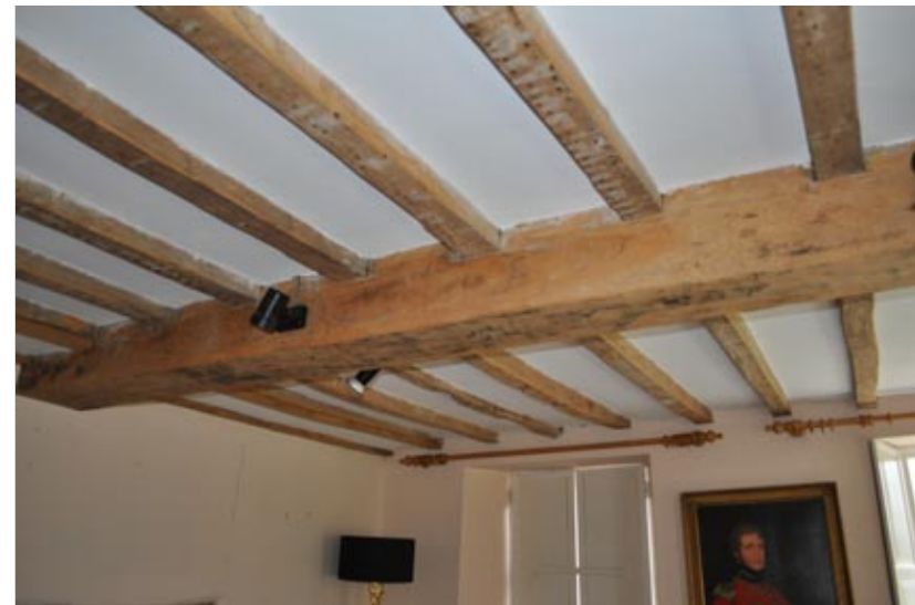
Plate 17. Living room, phase 3, ceiling details
