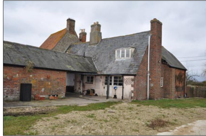
Plate 3. East & south elevations of Pound Farm
