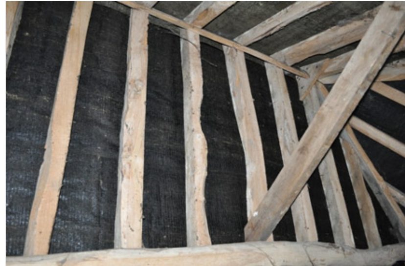
Plate 33. Rafters in attic, west wing
