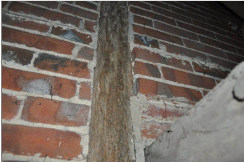
Plate 32. Timber framing in attic, west wing
