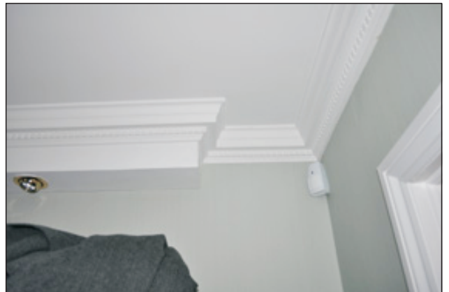
Plate 19. Phase 2b evidence of earlier chimney
