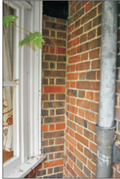
Plate 10. Phase 5 (left) butting Phase 2b (right)
