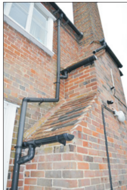
Plate 14. Detail of northeast chimney butted to Phase 2b structure
