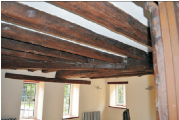
Plate 5. Phase 1b internal ground floor
