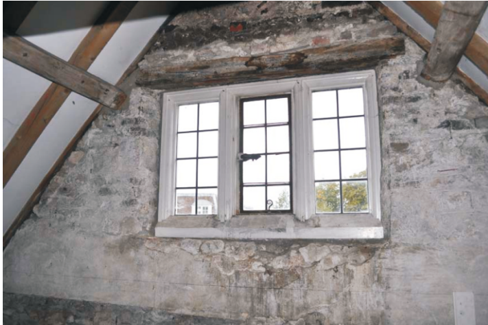
Plate 6: Mullioned window in attic
