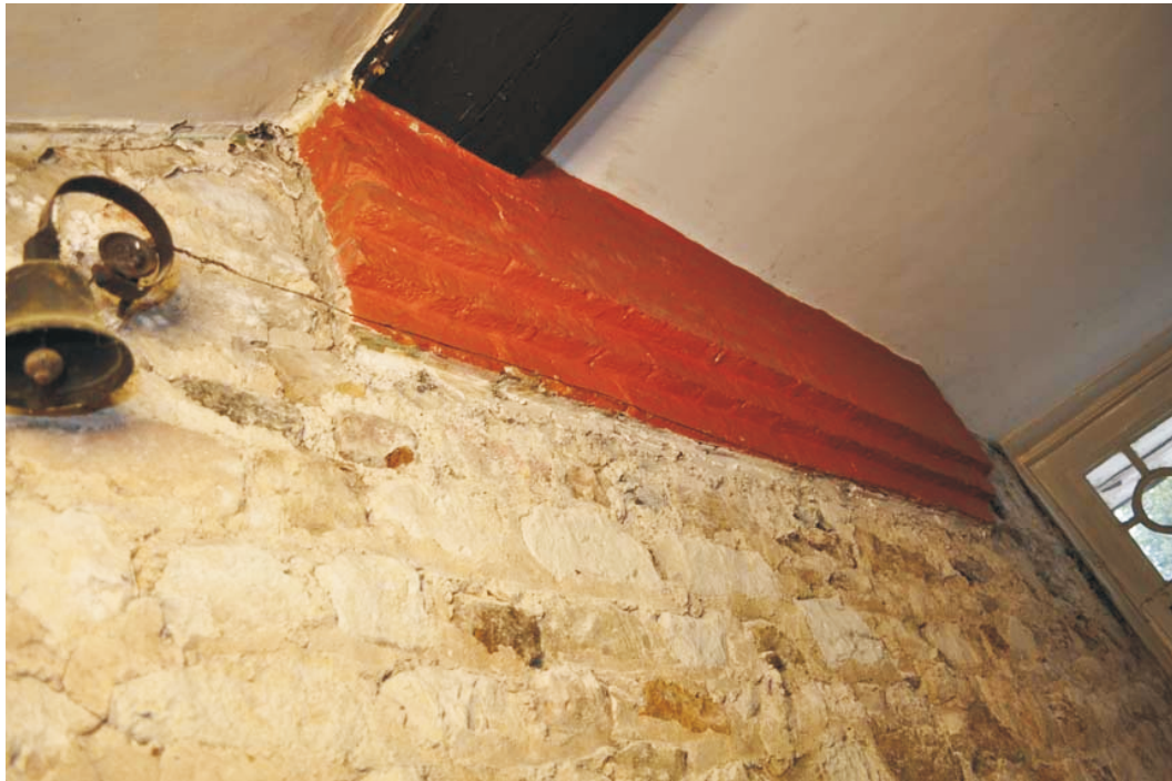
Plate 9: Projecting first floor chimney, originally external feature
