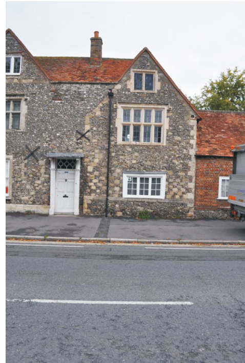
Plate 2: Gable of East Wing
