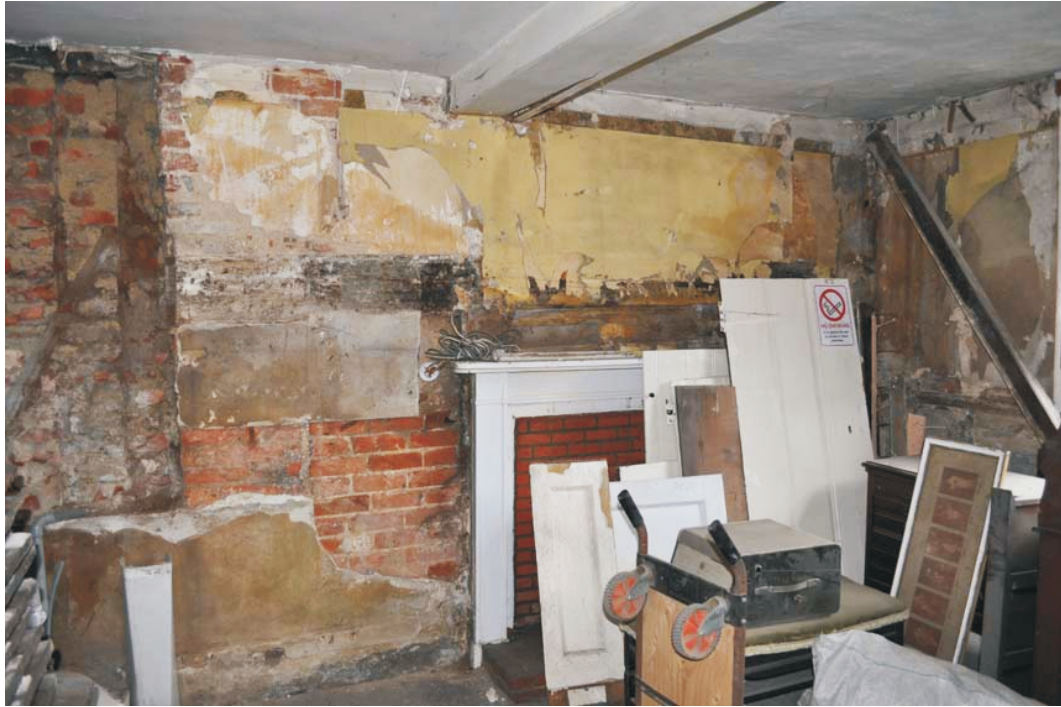
Plate 4: Blocked up fireplace at rear of building
