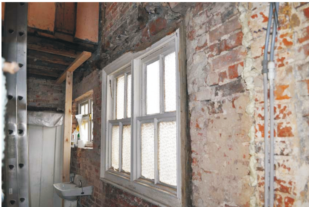
Plate 3: Butt in back wall between East Wing and back wall
