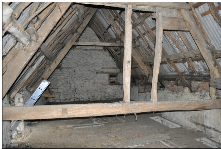
Plate 16. Building 4, west component loft
