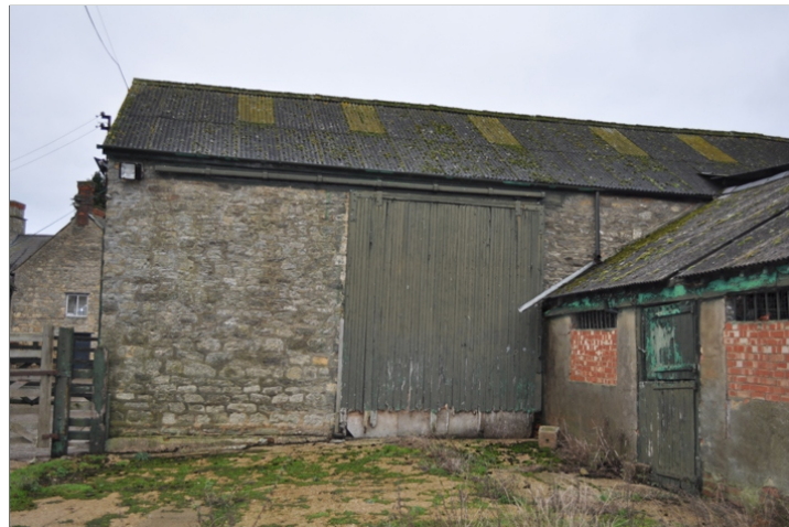
Plate 6. Building 2, east facade
