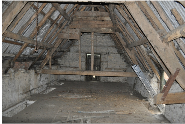
Plate 15. Building 4, west component loft
