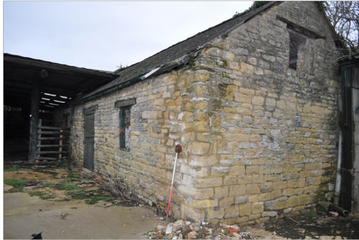
Plate 19. Building 3, south and west facade
