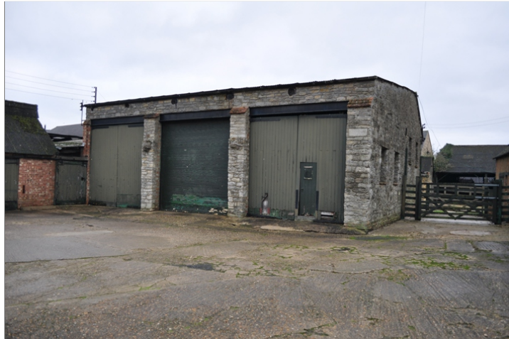
Plate 4. Building 2, west facade
