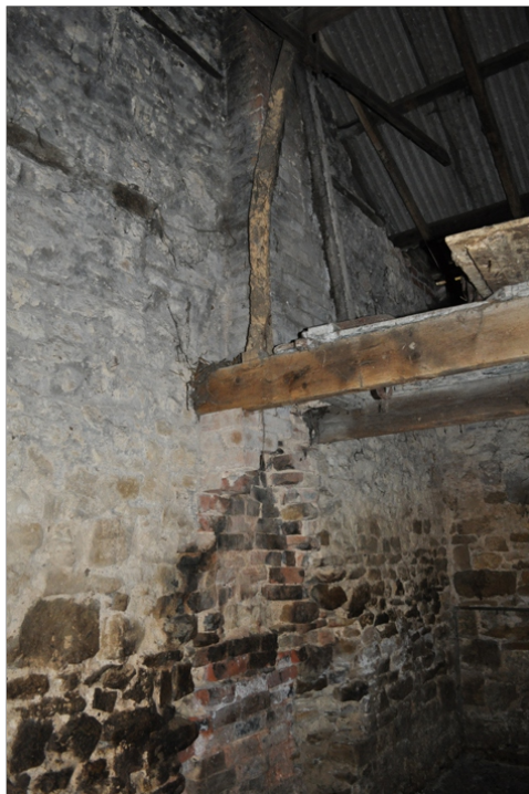
Plate 17. Building 4, east component
