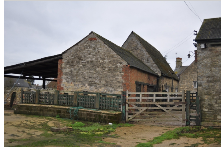
Plate 12. Building 4, north and east facade
