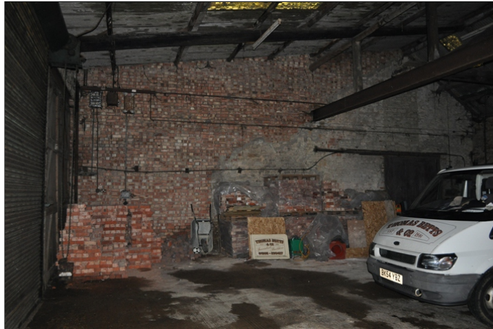
Plate 8. Building 2, Component B internal
