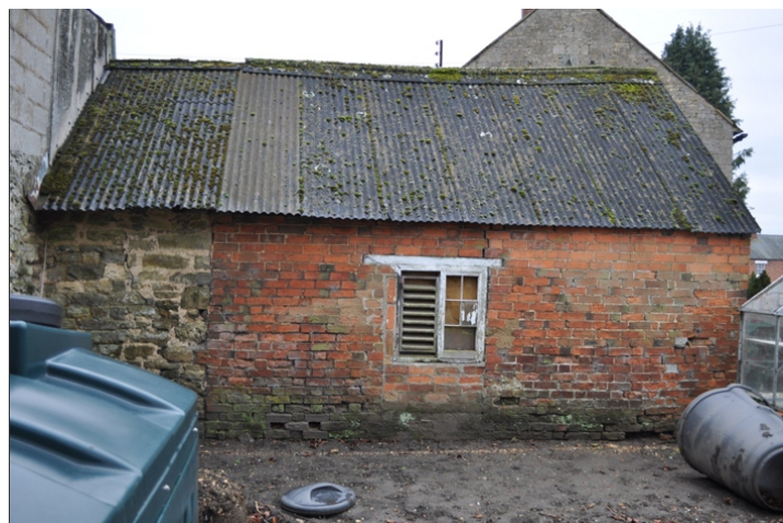
Plate 3. Building 1, north facade
