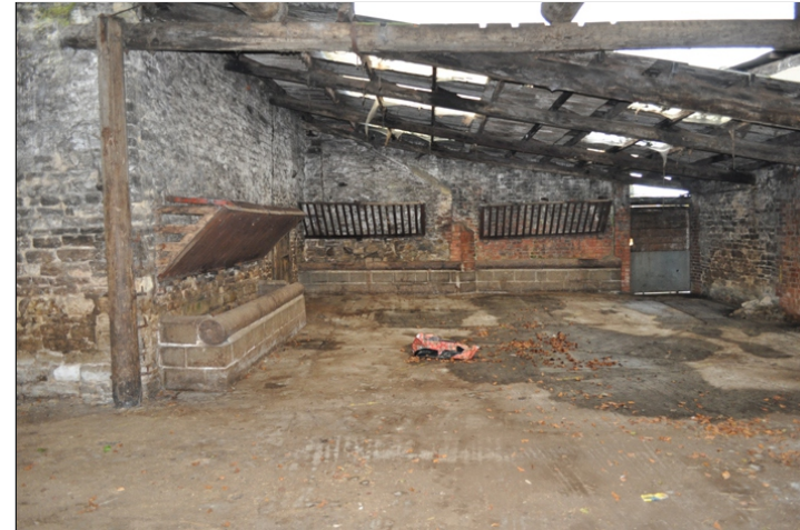
Plate 5. Building 2, north facade
