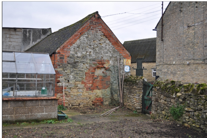
Plate 2. Building 1, east facade
