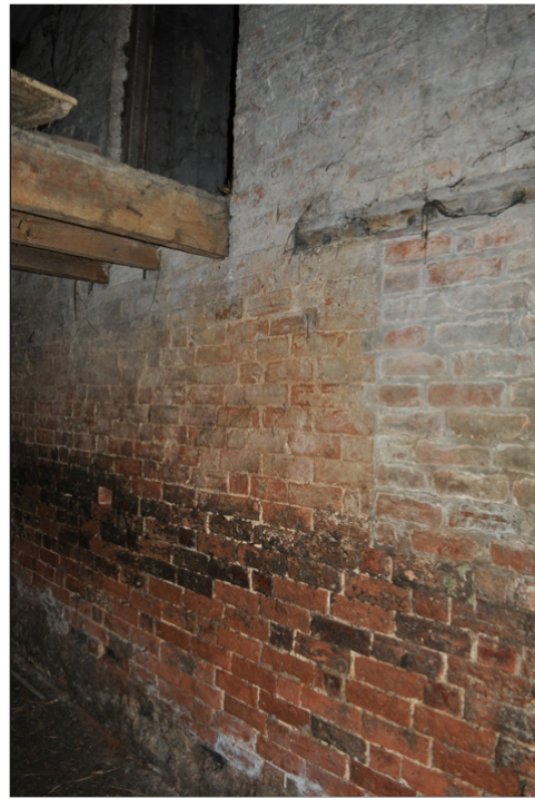
Plate 18. Building 4, east component
