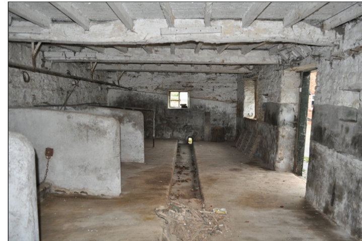
Plate 14. Building 4, west component ground floor
