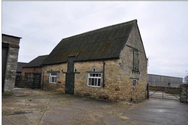
Plate 11. Building 4, north and west facade
