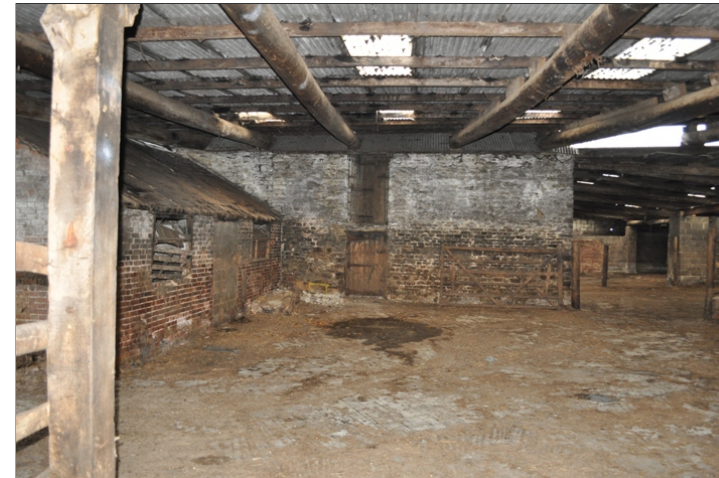
Plate 7. Building 2, east facade
