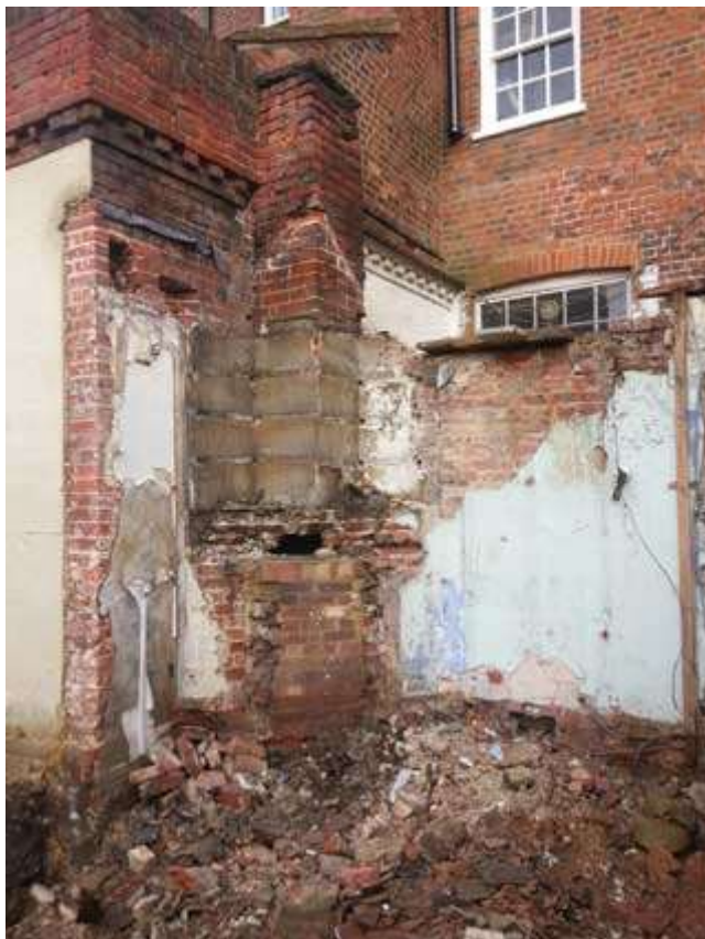
Plate 6 RE2 chimney and fireplace
