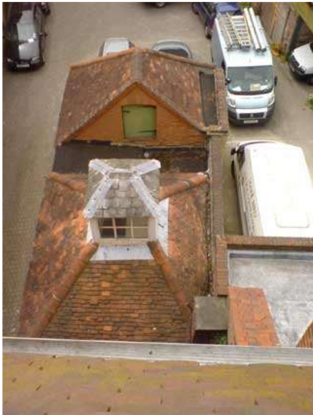
Plate 3 Kitchen wing roofs
