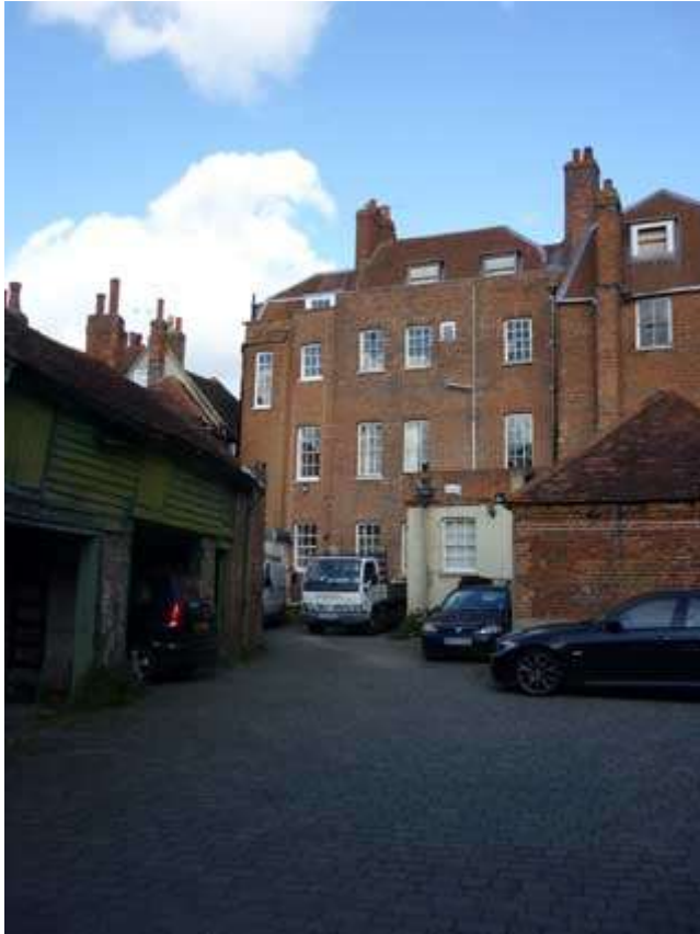
Plate 4 Part of the rear façade
