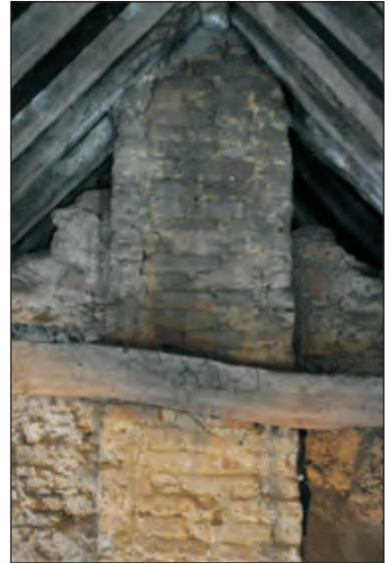
Plate 8. Detail of chimney to be removed.
