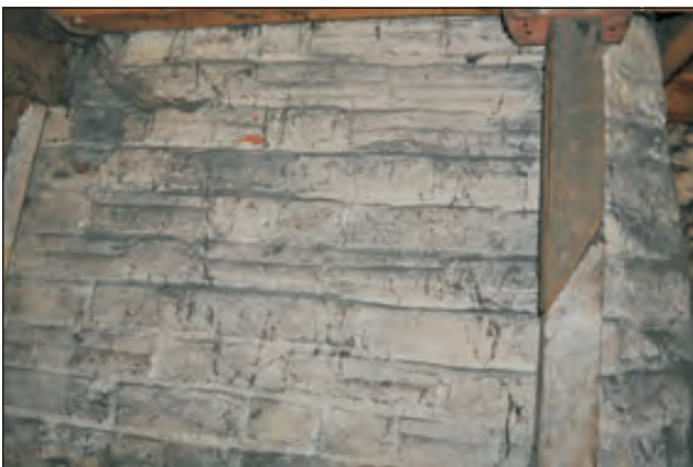
Plate 10. Detail of chimney to be removed.
