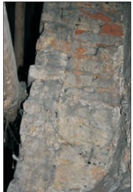
Plate 11. Detail of chimney to be removed.
