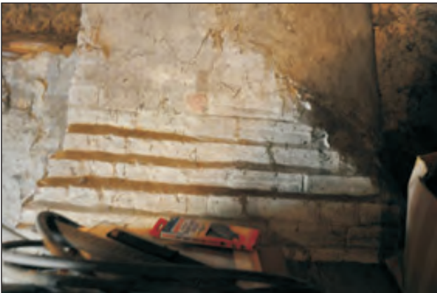
Plate 9. Detail of chimney to be removed.
