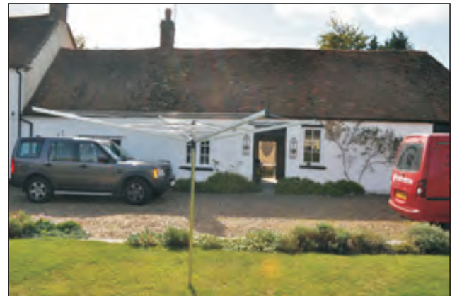
Plate 4. North elevation of barn.
