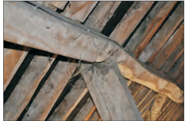
Plate 15. Roof features in barn.
