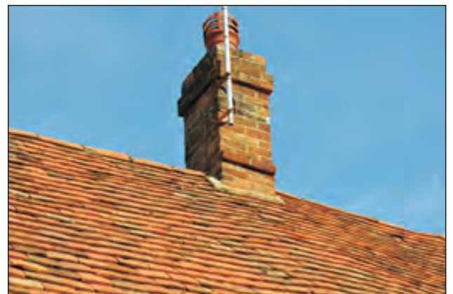
Plate 6. Chimney located along the line of roof of the barn.
