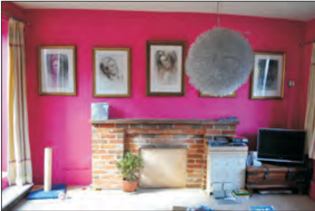
Plate 7. Internal fire place to be removed.
