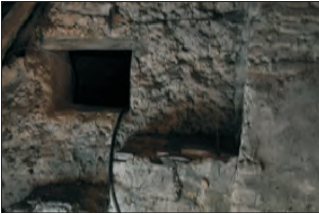
Plate 12. Details of wall between barn and house.
