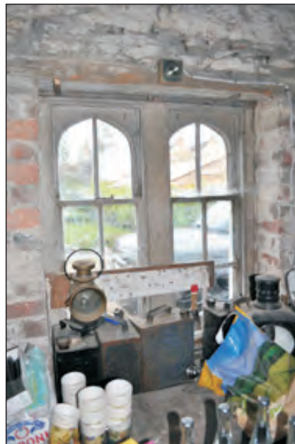
Plate 16. Window details in barn.
