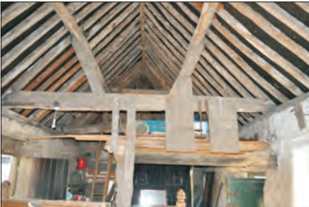
Plate 14. Roof features in barn.
