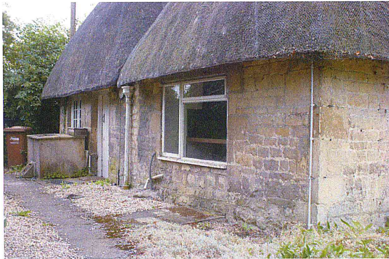
Plate 3: The east elevation of Hillside Cottage.
