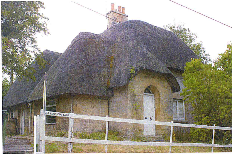
Plate 1: The north elevation of Hillside Cottage.
