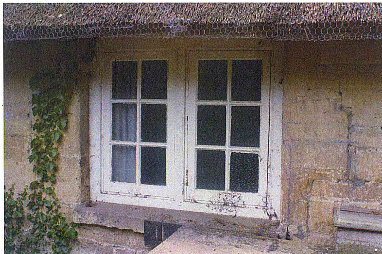
Plate 6: The bathroom window which has possibly been reset.
