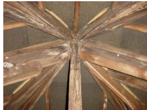
Plate 8: Apex Detail of King-post in hub roof
