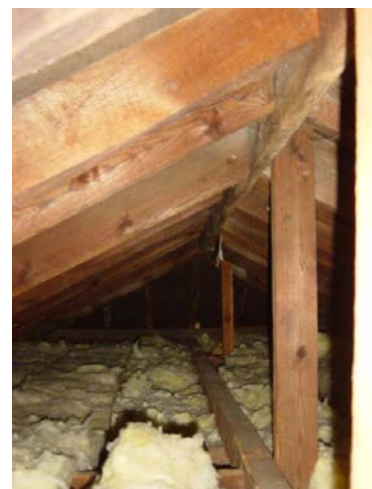
Plate 10: Vertical supports in West Wing roof construction
