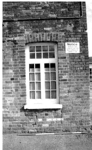
Plate 22: Blocked door in west elevation of East Wing
