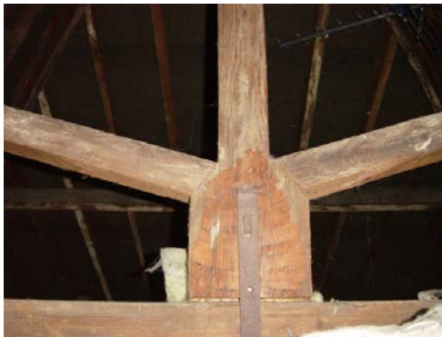
Plate 7: Base Detail of King-post in hub roof
