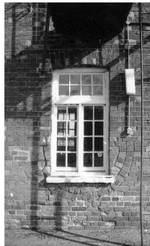
Plate 23: Relieving arch in west elevation of East Wing truncated by inserted Type 4 window
