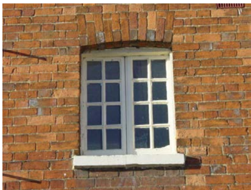
Plate 1: Type 2 Window with Vitrified Headers
