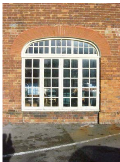
Plate 4: Type 3 Window with Gauged Brick Basket Arch
