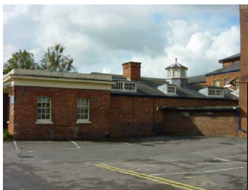
Plate 15: General View of Kitchen Range and junction with hub (arrow points to small window at apex of kitchen roof where it meets the hub)
