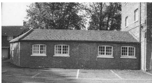
Plate 29: Southwest Range, eastern elevation
