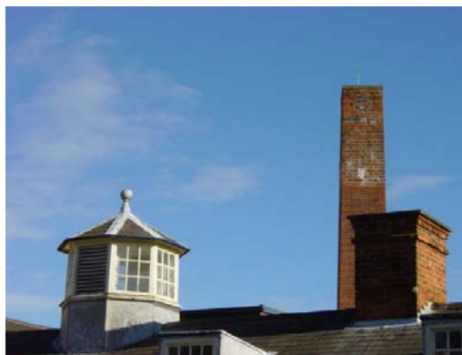
Plate 11: Kitchen Range roof lantern and chimney
