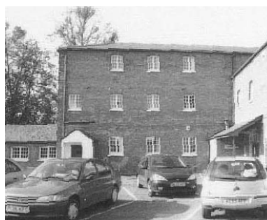
Plate 36: In situ original windows and largely un-altered fenestration (east elevation of West Wing)
