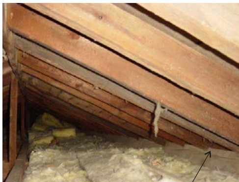
Plate 9: Birdsmouth detail in West Wing Roof Construction
