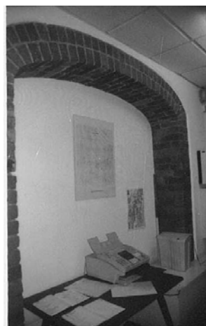
Plate 24b: Blocked arch access from West Wing to Spoke
