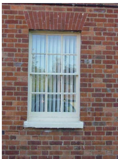
Plate 3: Type 1 Window with Gauged Brick Arch
