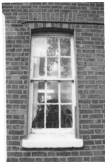
Plate 33: Inserted Type 1 window in west elevation of West Wing
