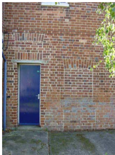
Plate 27: Blocked doorway and later inserted door in window opening of Northeastern Range
