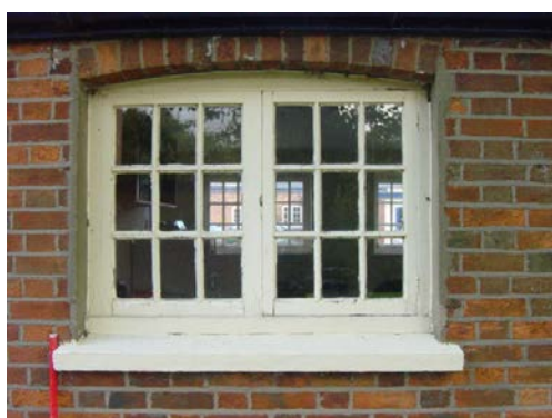
Plate 31: Inserted window in west elevation of Southwest Range
