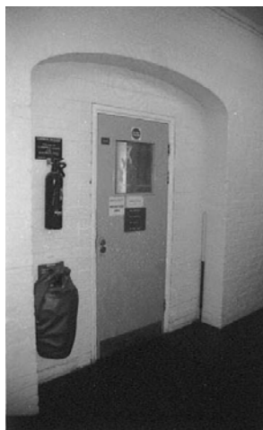
Plate 24a: Partially blocked arch access from East Wing to Spoke
