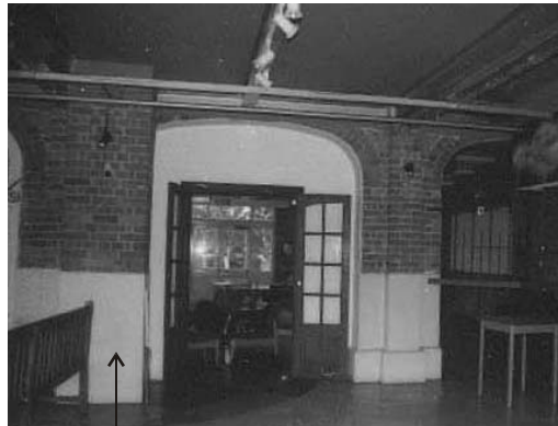
Plate 6: Inserted Chimney in East Spoke (Truncates original arch)
