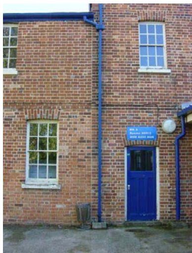
Plate 26: Straight Line Join (SLJ) between East Wing and later Northeastern range
