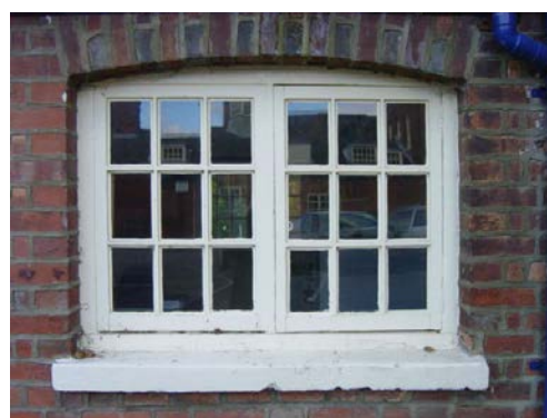
Plate 32: Replaced window in original opening on eastern elevation of Southwest Range
