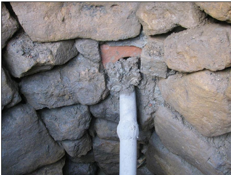
Plate 7: Post-medieval modification to well 4. Looking west.
