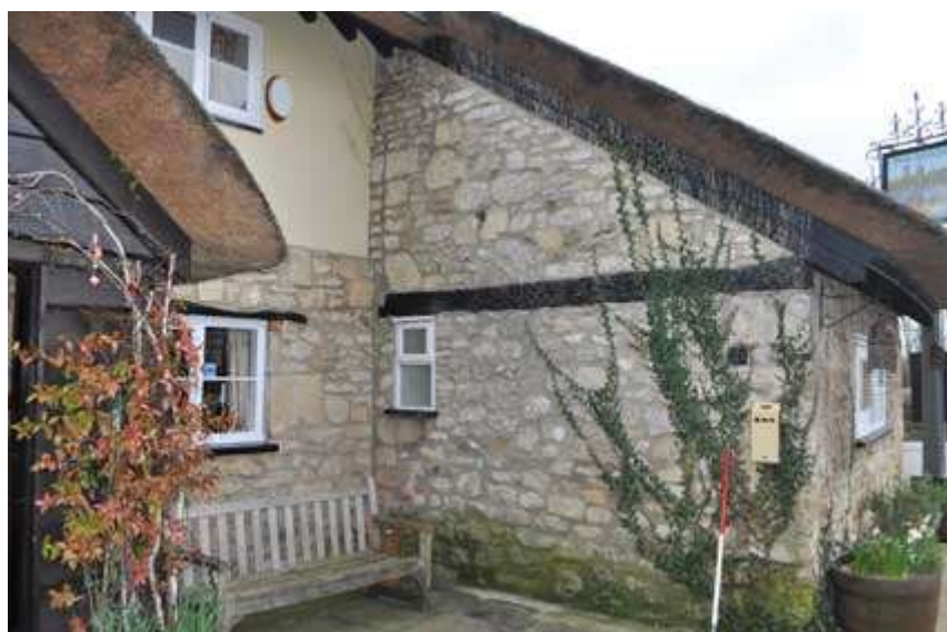
Plate 12 Butt joints of Phase 3
