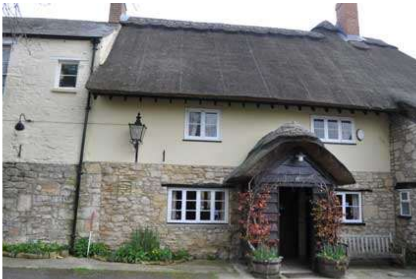
Plate 1 Old southwest façade
