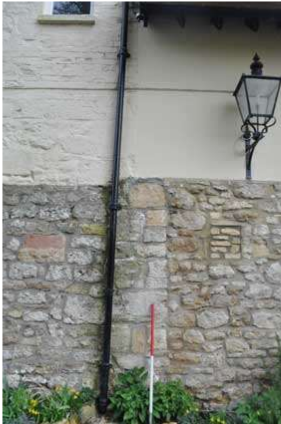
Plate 13 Butt joint for north extension
