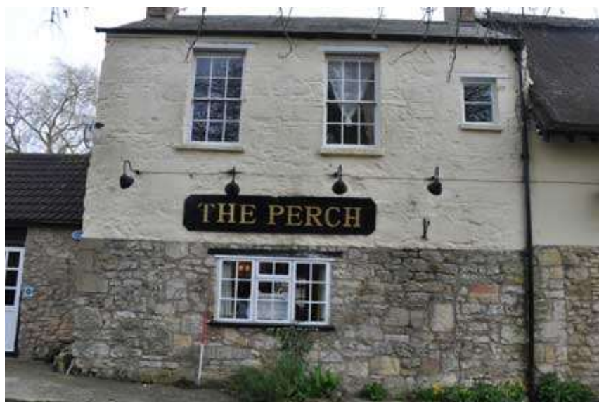
Plate 2 Northern extension southwest façade
