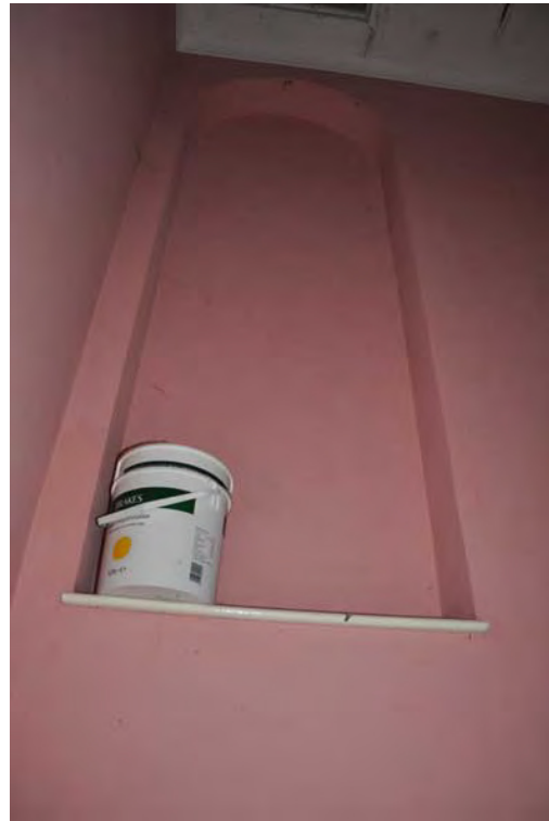
Plate 19. Details above back stairwell
