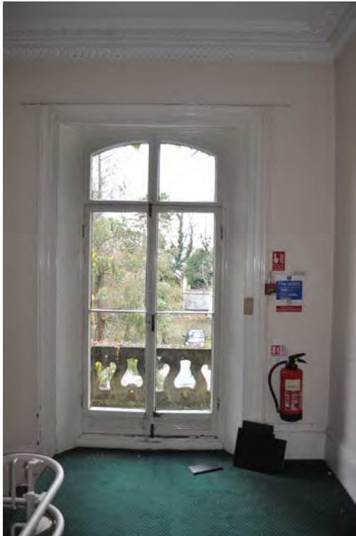
Plate 15. First floor landing details
