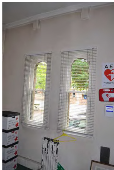
Plate 14. Details ground floor northeast room
