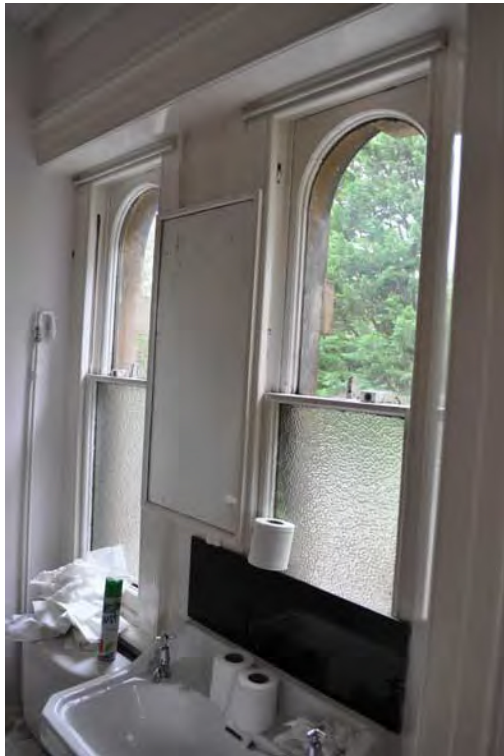
Plate 18. First floor details east side central room
