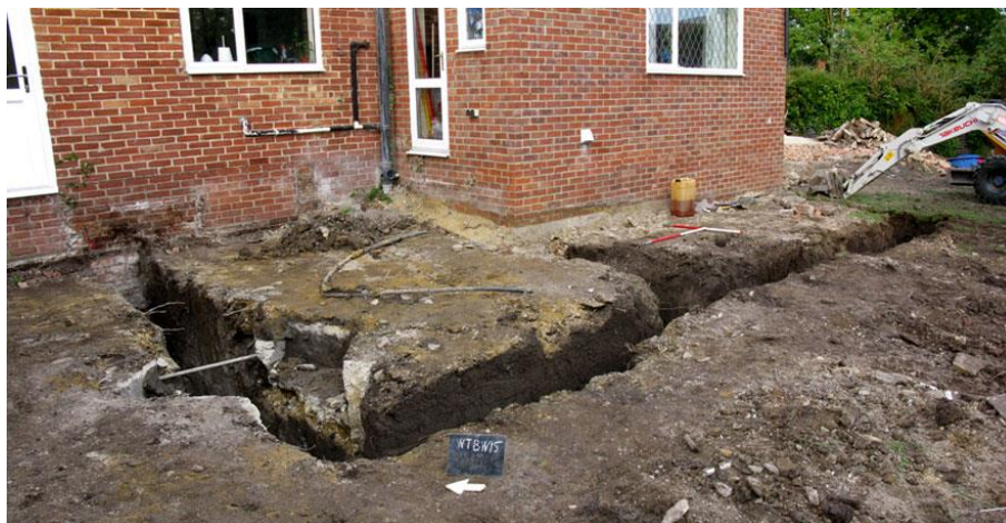
Plate 1: General overview of foundation trenches, looking NE
