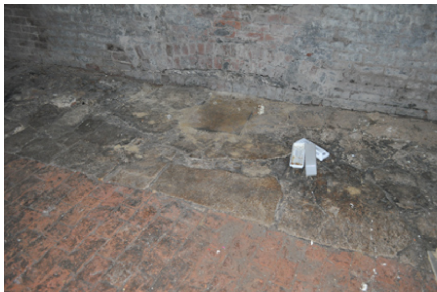
Plate 14: Floor in basement (B1)
