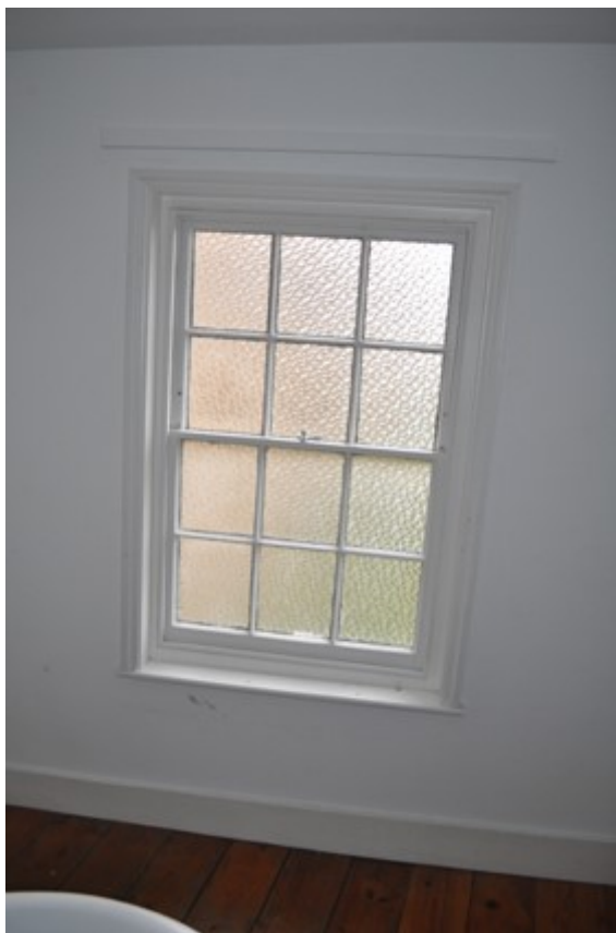
Plate 22: Sash window in F2
