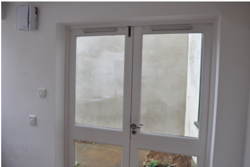
Plate 18: Internal view of east wall in G2
