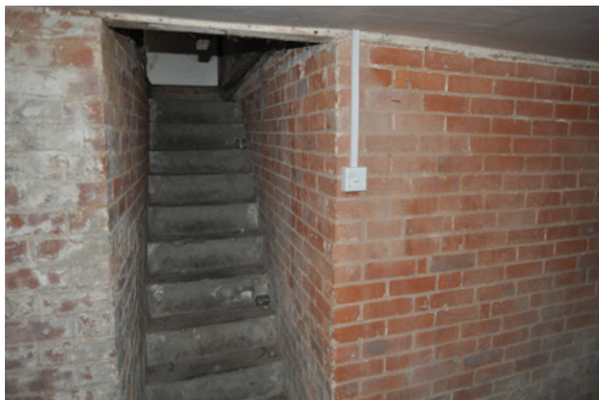
Plate 26: Staircase in Basement
