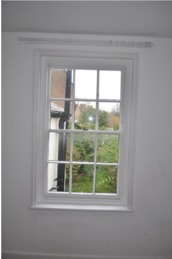
Plate 9: Sash window in bedroom 1 (F3)
