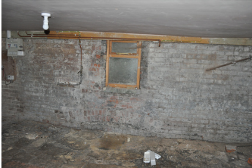
Plate 12: Window and segmental arch in basement (B1)
