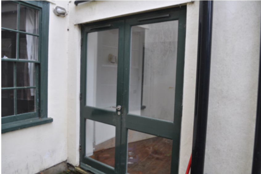
Plate 17: External view of east and south wall
