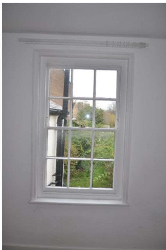
Plate 23: Sash window in F3
