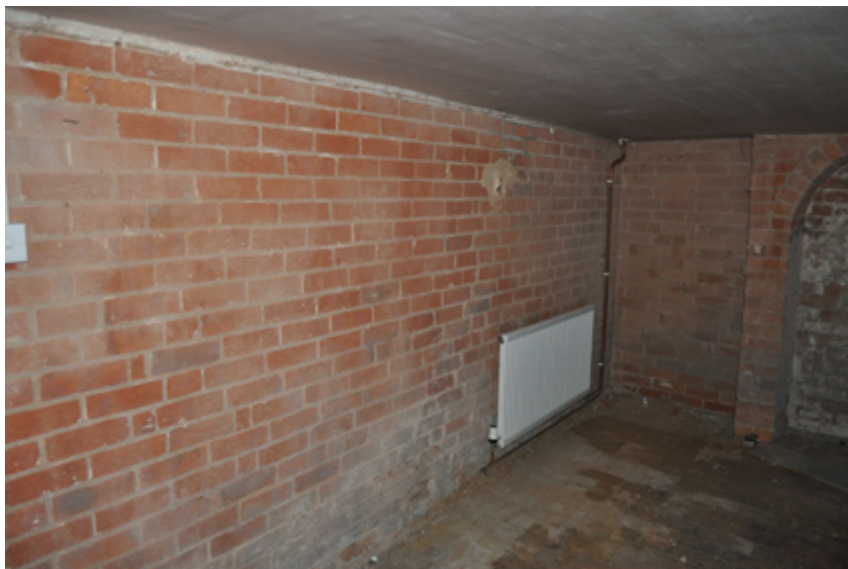
Plate 25: East wall in Basement
