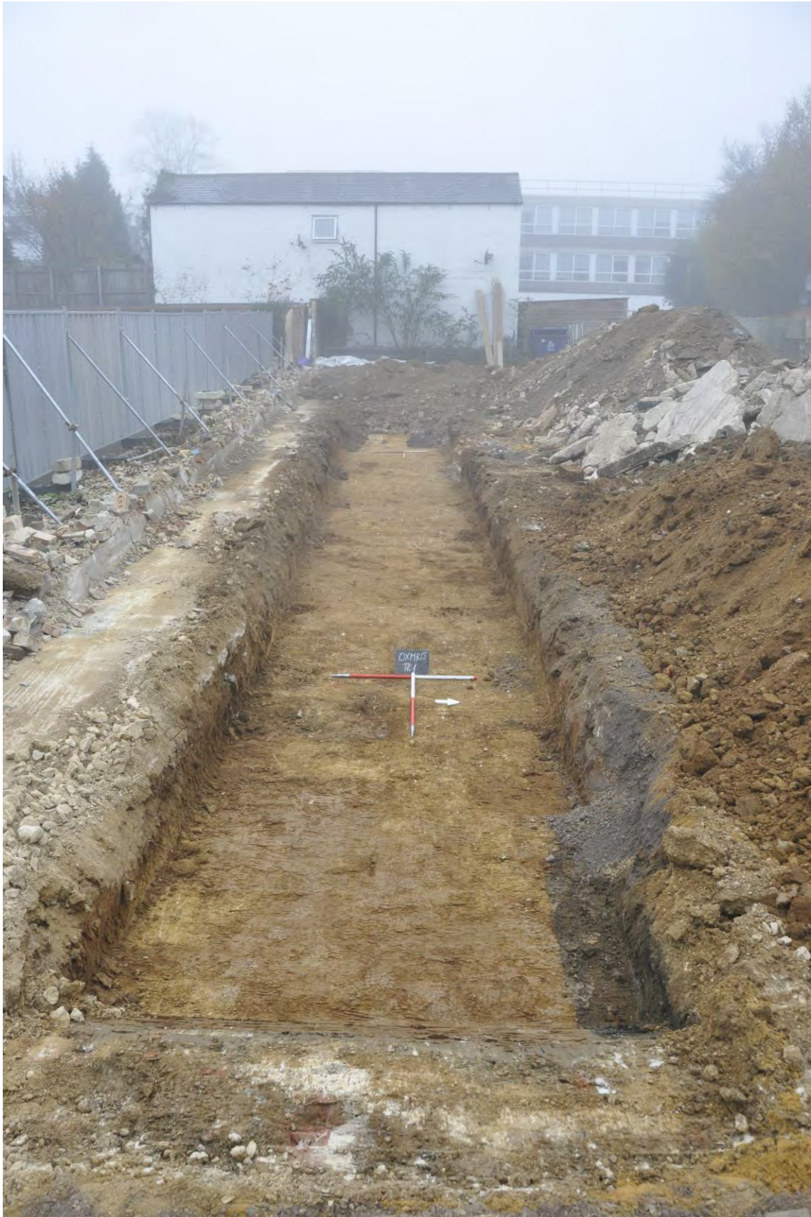
Trench 1. View to west.
